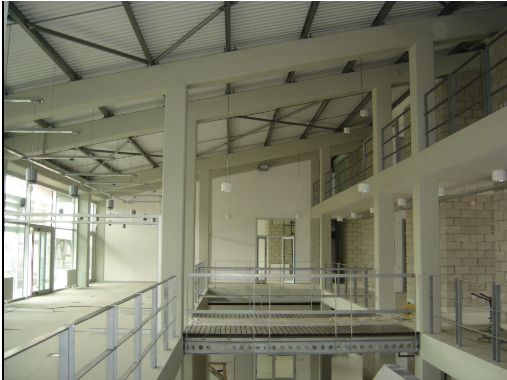
Figure C.4 MATPUM Building Inner View
