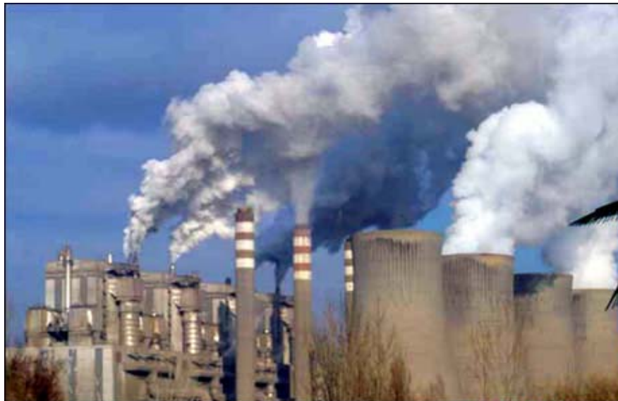
Figure 2.1 Exhaust Gases Pouring out from Conventional Plants
