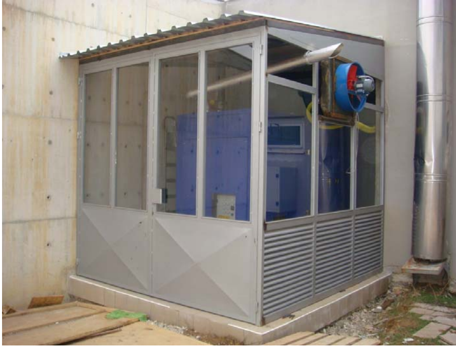
Figure D.7 ICE After the Construction- Outside View
