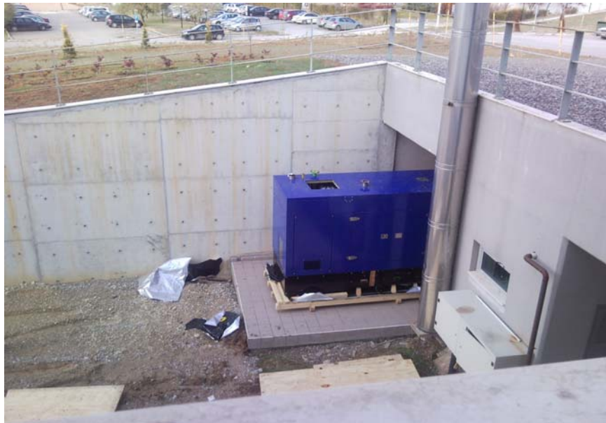
Figure-D.4 HEGEL ICE Co-generator
