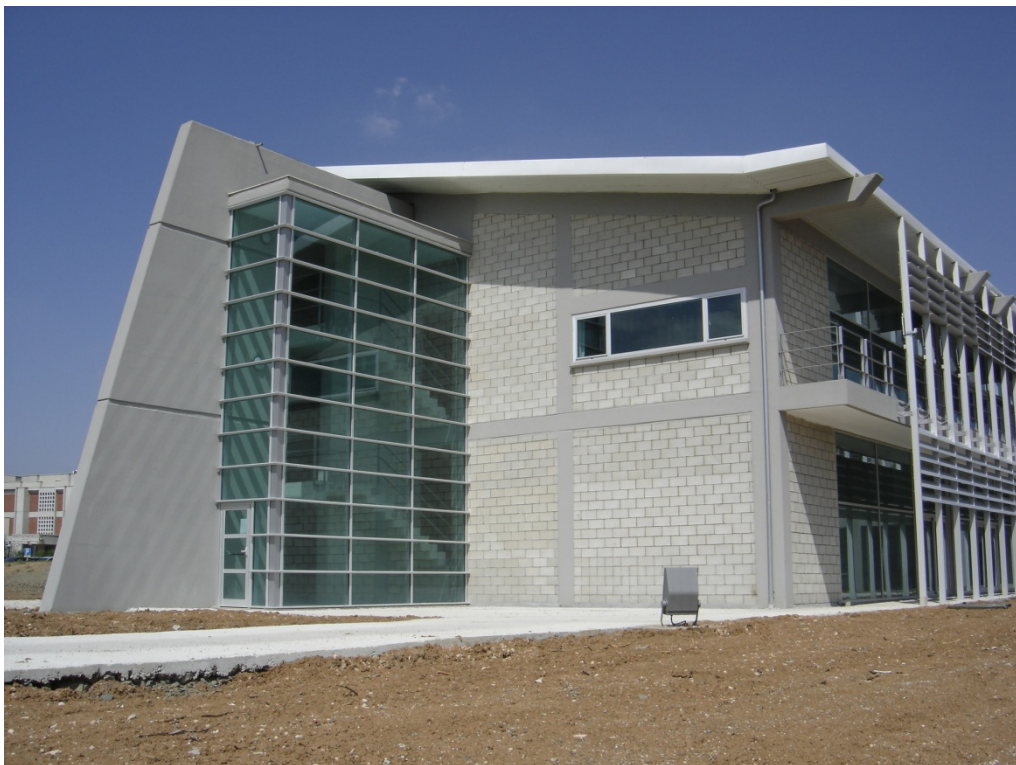
Figure C.3 MATPUM Building, Side View
