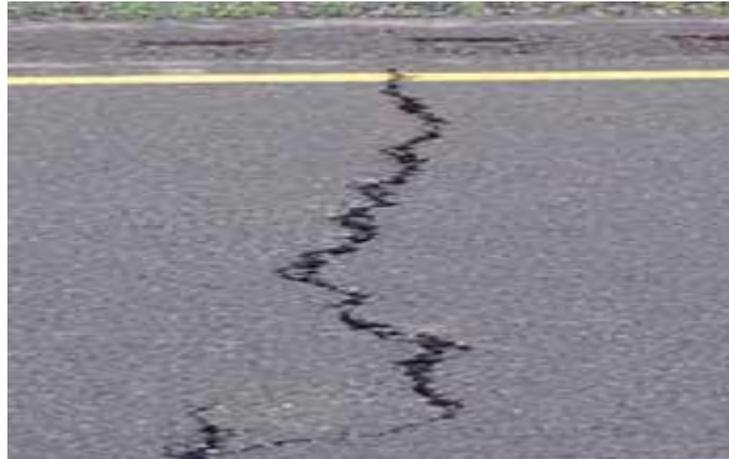
**Figure 2.2- A view of low temperature cracking on an AC pavement section (Transport Pooled Fund Study 776, 2007)**
