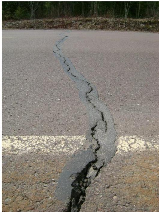
**Figure 2.5- An example of a low temperature cracking in AC pavements**
