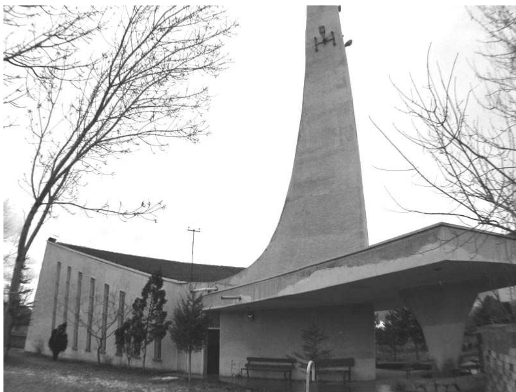
Figure 70. North and East facades, Derinkuyu Mosque (Photograph by Özgür Ürey)
