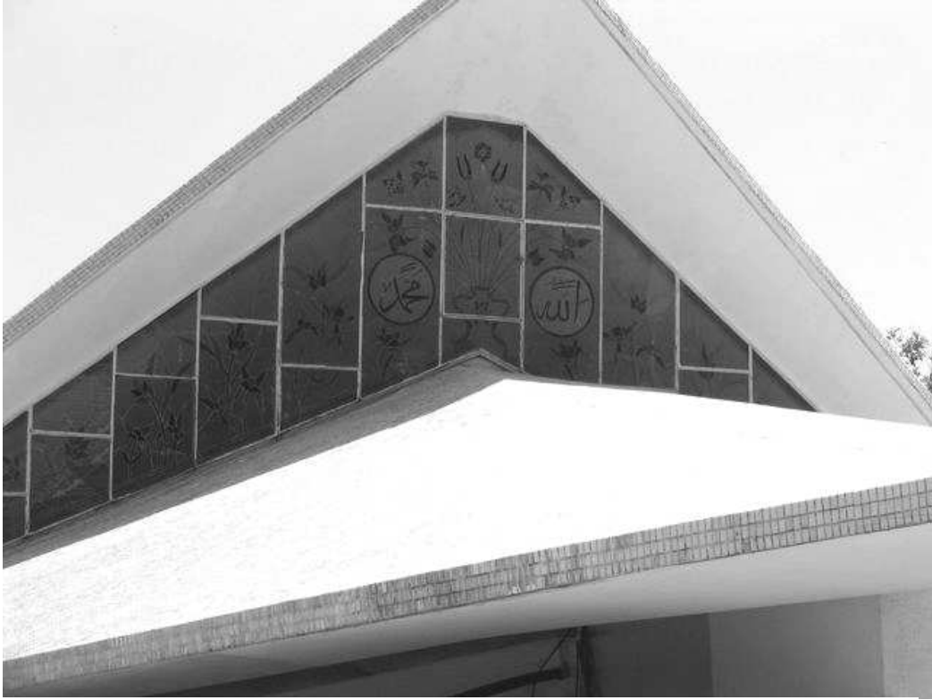
Figure 26. Roofing from exterior, Kınalıada Mosque (Photograph by Özgür Ürey)
