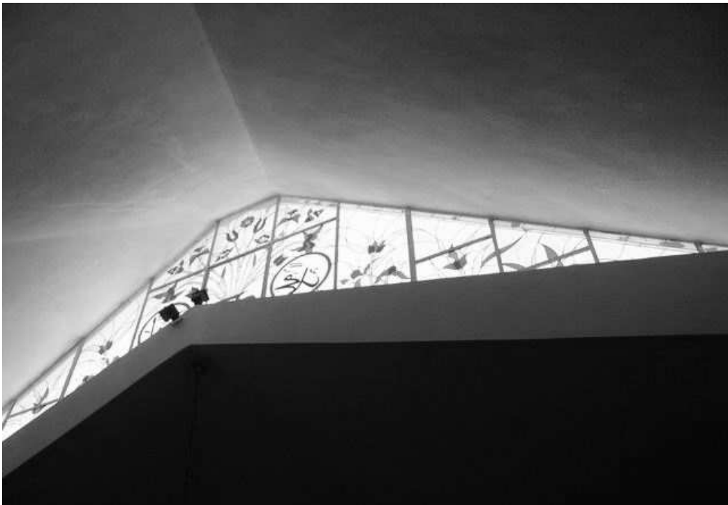
Figure 27. Roofing from interior, Kınalıada Mosque (Photograph by Özgür Ürey)
