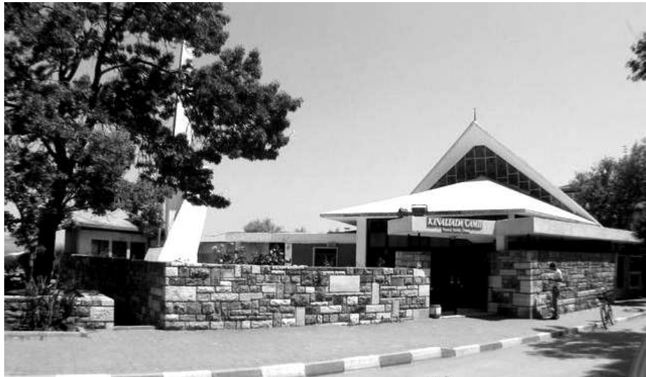
Figure 15. Main entrance, Kınalıada Mosque (Photograph by Özgür Ürey)
