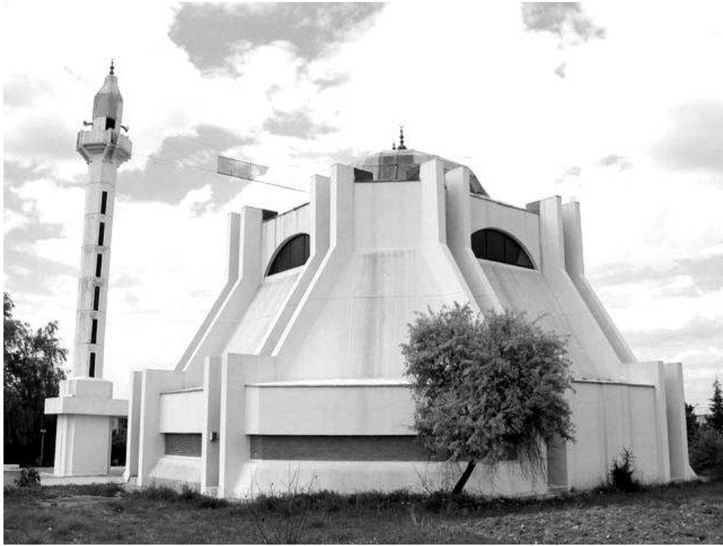
Figure 34. South and west wall, TEK Mosque (Photograph by Özgür Ürey)
