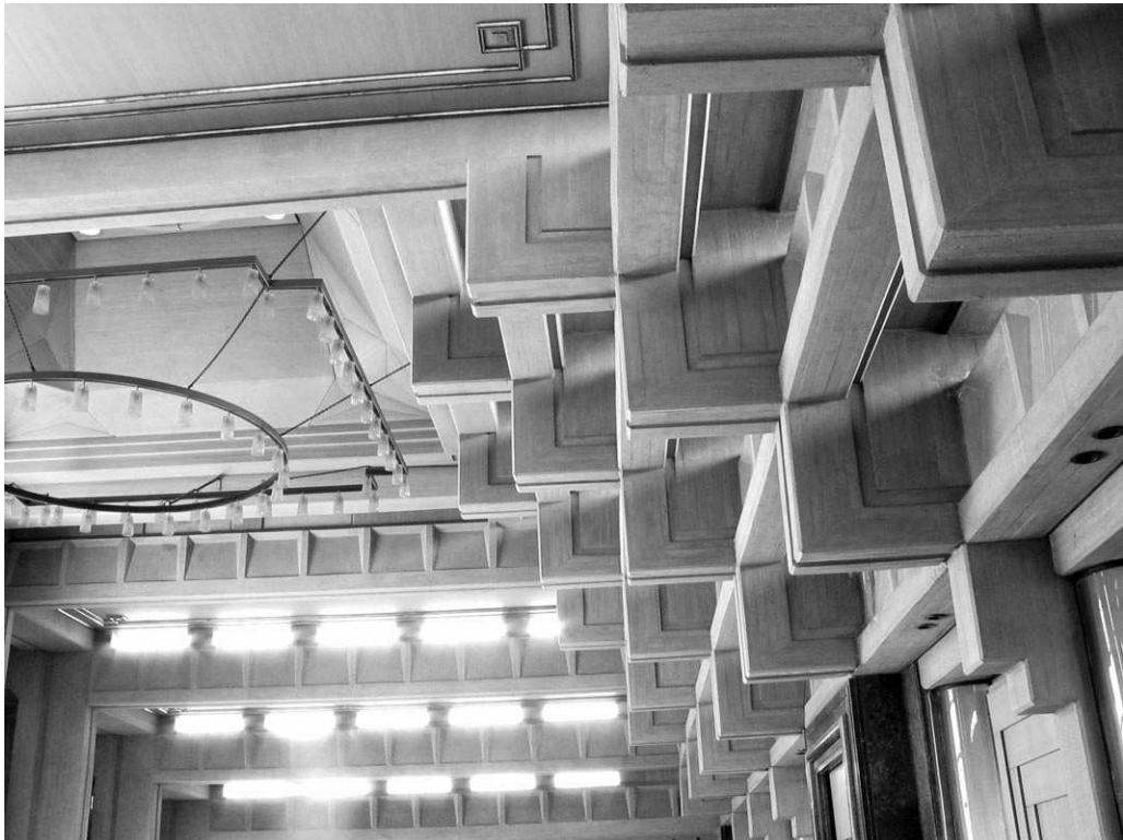
Figure 46. Roof structure from interior, TBMM Mosque (Photograph by Özgür Ürey)
