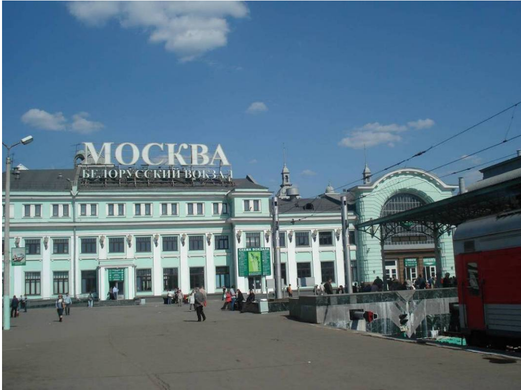
Figure 50 Platform of Belorussky Railway Station. (Author 06.2009)
