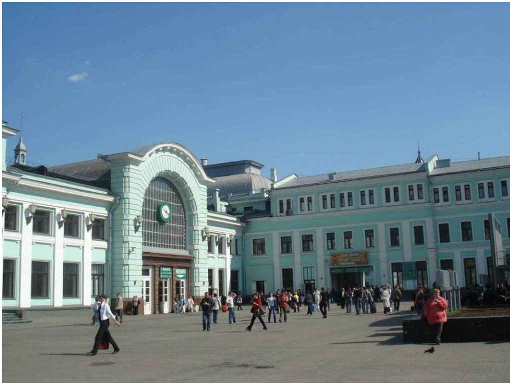
Figure 51 Platform of Belorussky Railway Station. (Author 06.2009)
