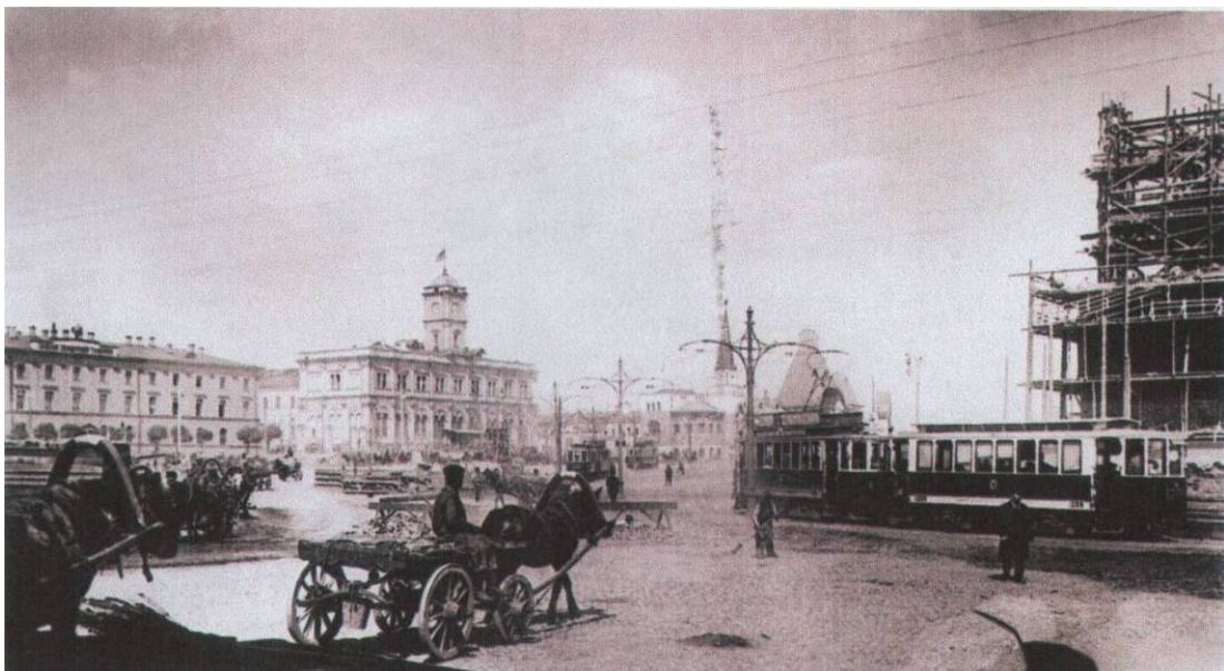
Figure 36 Kazansky Railway Station under construction. (Museum of History of Moscow)
