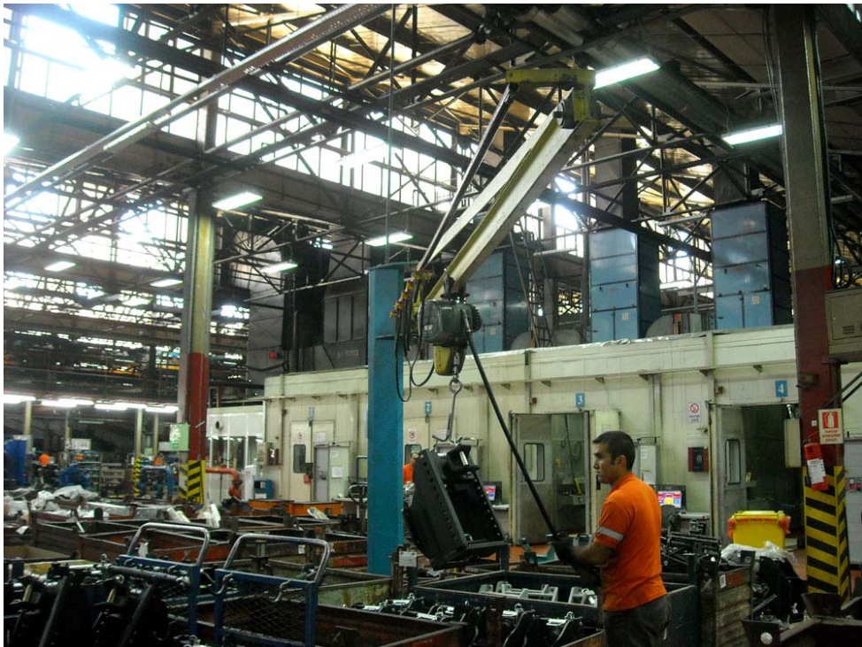
Figure A.7: The remote controlled system carrying the engines or gear boxes to the desired point.
