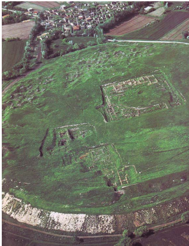
Figure 4.6. View of the mound of Kültepe, showing the monumental buildings and the surrounding Hellenistic and Roman fortification wall. (After T. Özgüç 2005.) Özgüç (1999, 73) states that in the investigated part of the wall, there is evidence for the underlying early fortification wall.
