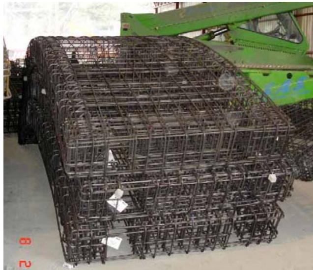
Figure 2.13. Typical reinforcement cage for segmental linings
