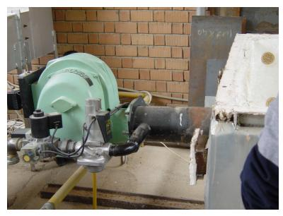
Figure 3.9 Alarko Lamborghine Natural Gas Burner
