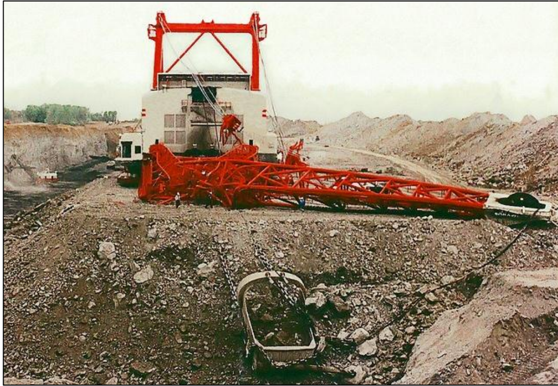
Figure 2.4 Dragline Boom Failure (Davis, 2010)
