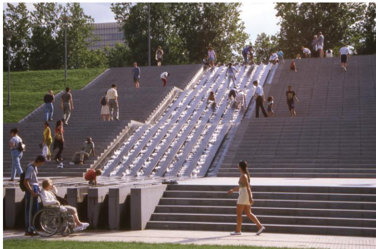
Figure 37. View of Bercy Park showing the connection stairs to the Grand Terrace. Photograph is taken from the personal archive of Căna Bilsel.
