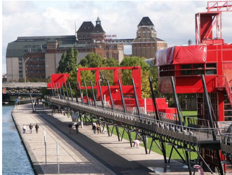
Figure 15. View of Parc de la Villette showing the gallery and the folies. Per Wahlin, "Cable-stayed Bridges of Europe," http://www.pwpeics.se/images/pw%20cs/france%20p-z/Paris_La_Villette2.JPG (accessed December 6, 2010).
