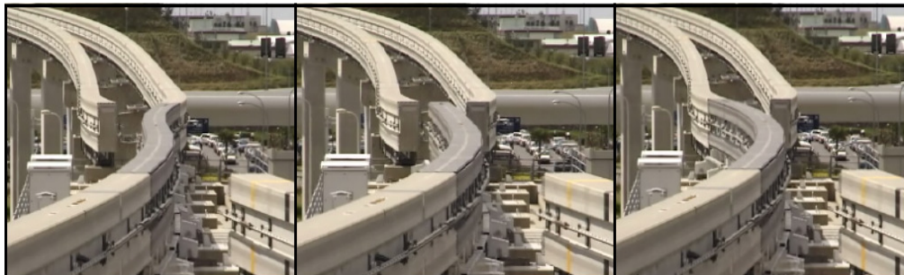
Figure 3.10: Flexible monorail switching system in three different situations ( www.hitachi-rail.com , last accessed on 10/10/2010)
