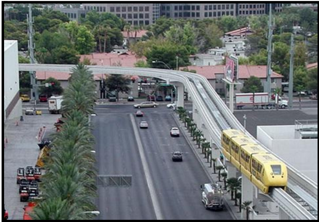
Figure 3.14: Las Vegas Monorail, Nevada, USA
