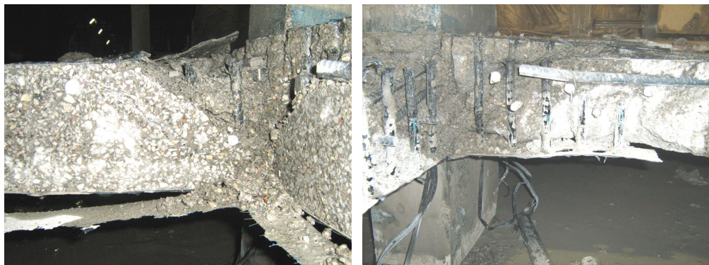
b) Inclined shear crack
