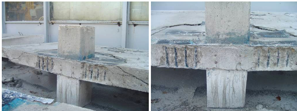
b) Inclined shear crack
