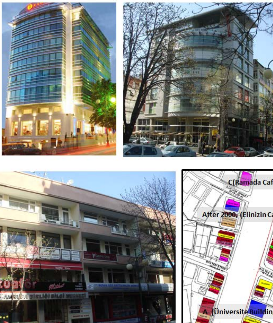
Figure 7-47, Dissimilar and interesting buildings on THS according to their architectural style (Resource: Personal study and rendering)
