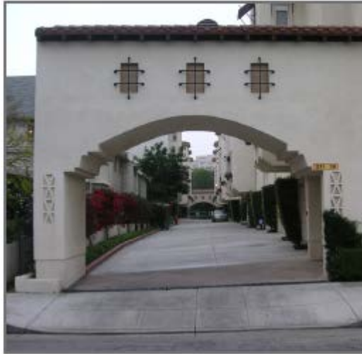
Figure 3-20, The use of architectural features to achieve a continuity between different parts of the pedestrian way (Resource: LA-Walkability Checklist, 2008, p.37)
