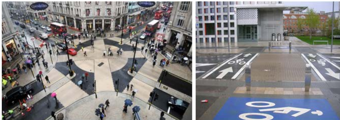
Figure 8-4, Safe street crossings with necessary traffic signage and textured pavement materials
