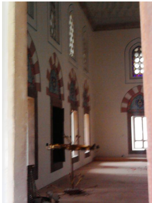
Figure 5.6 Photos of the applied restoration applications
