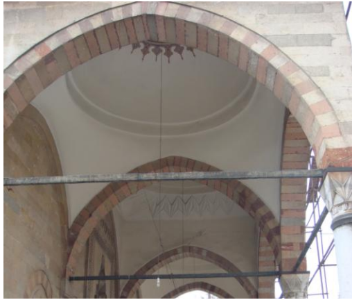
Figure 4.10 Photo of the structure's front section
