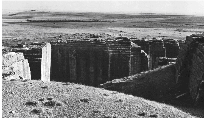
Figure 2.1 Quarrying stages of limestone on Walls of Dara (Thais, 2010)
