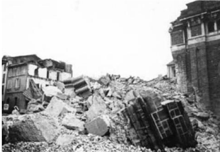
Figure 3.13 The ruins of The Civic Tower of Pavia after the collapse (Binda et al., 2008)
