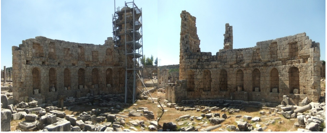
Figure 36. Inner façades of the courtyard walls (photos taken and edited by the author)
