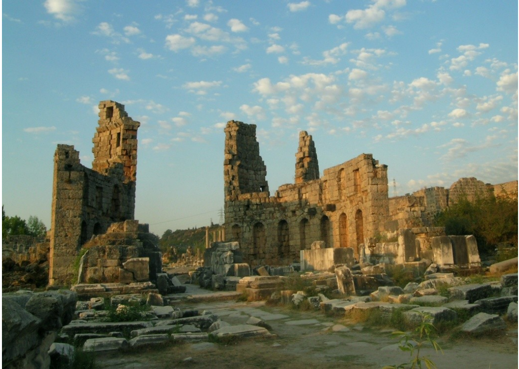
Figure 30. Hellenistic City Gate from north. The towers and the courtyard walls are still standing while the ceremonial arch and the arched gate between the towers are collapsed (photo by Ayşe Ercan)
