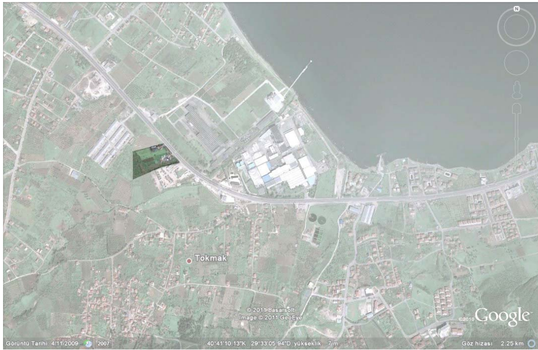
Figure 28 The plan of Karamürsel Temporary Housing Settlement showing the selection and planning considerations.
