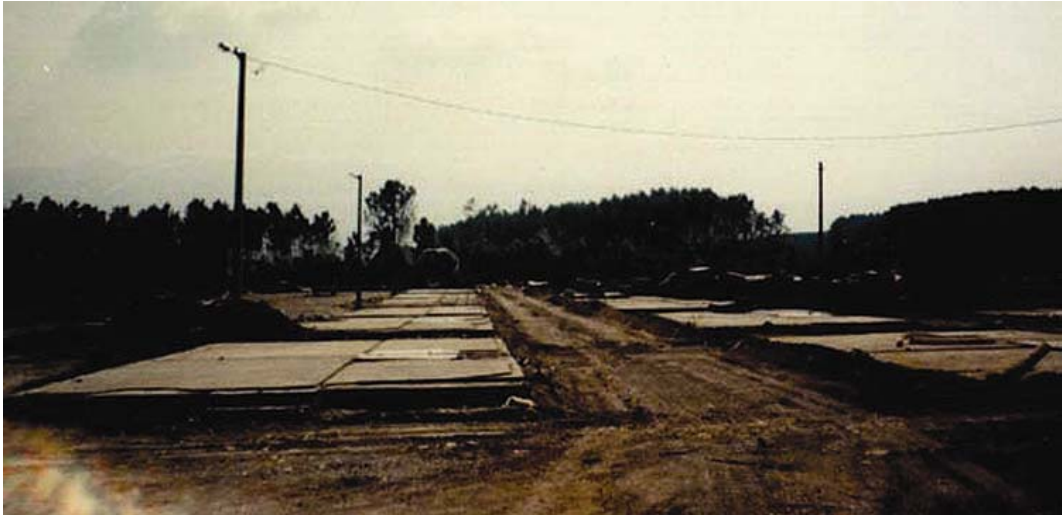
Figure 51 View of concrete foundations of temporary houses after dismantling.
