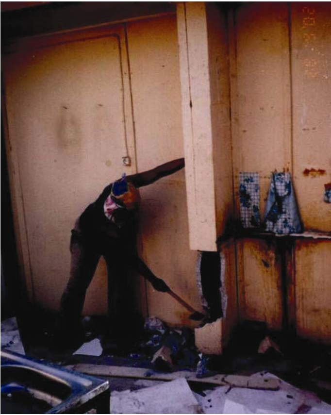
Figure 52 Dismantling operations carried out by subcontractors.
