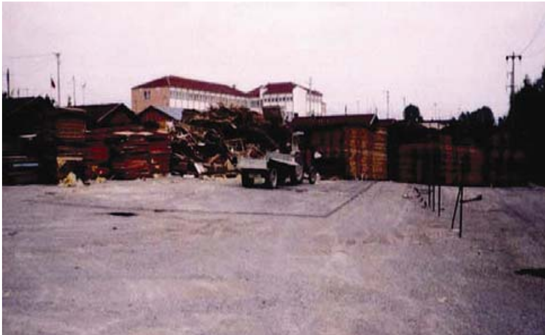
Figure 50 Inappropriate storage of sandwich panels of prefabricated houses.
