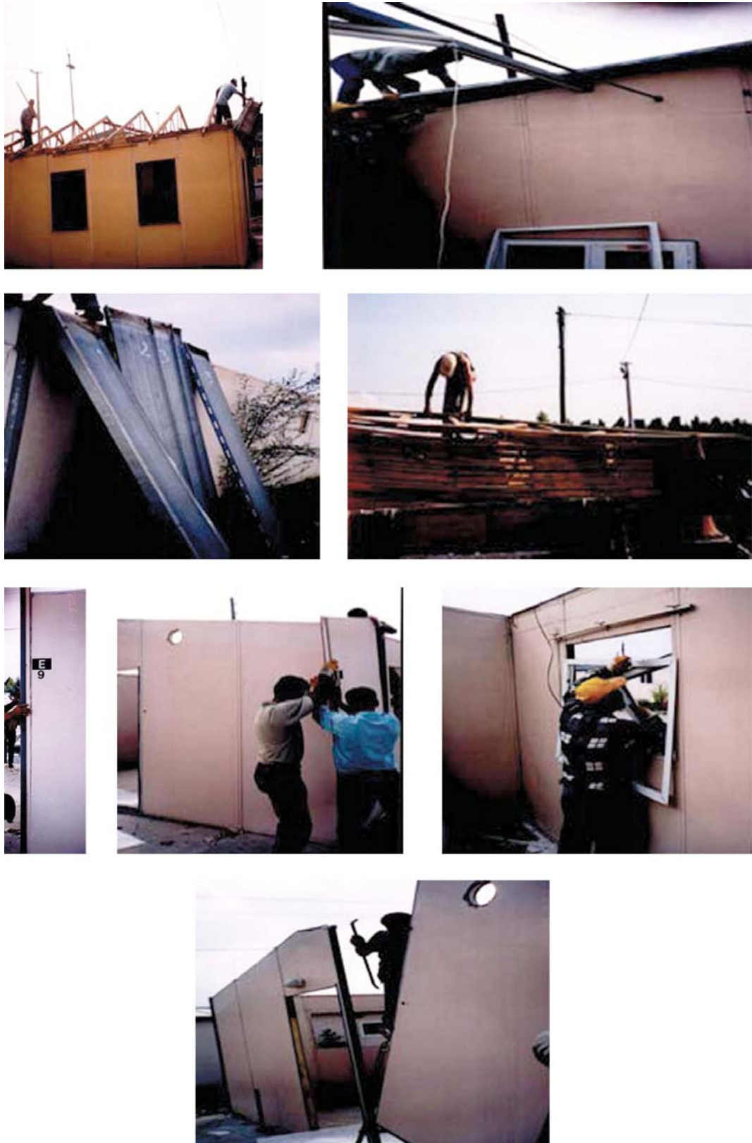
Figure 48 Dismantling steps of prefabricated houses in post-occupancy period.
