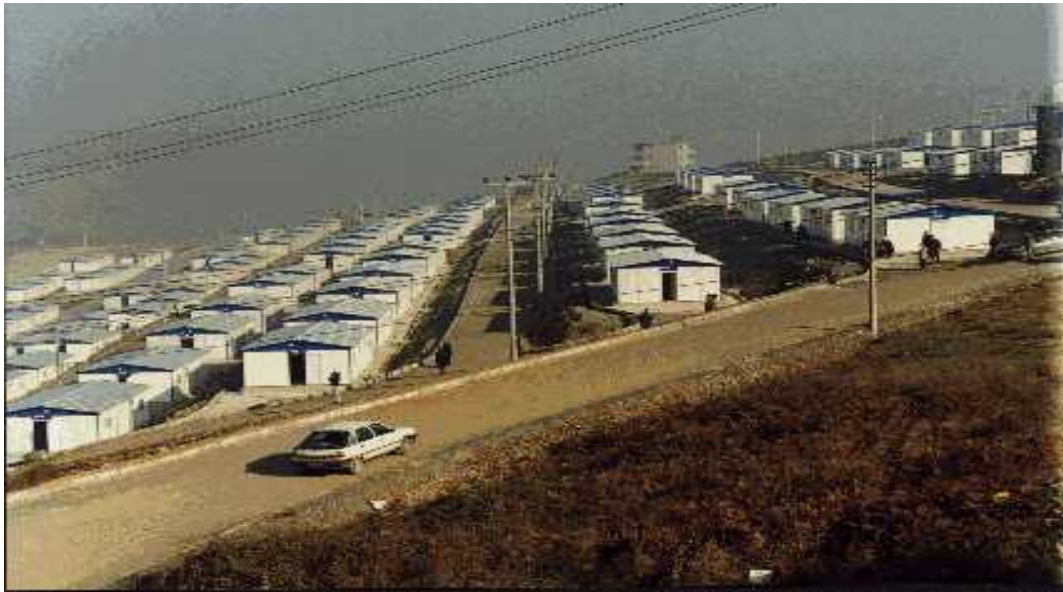
Figure 55 Prefabricated housing settlement in disaster area in 1999.
