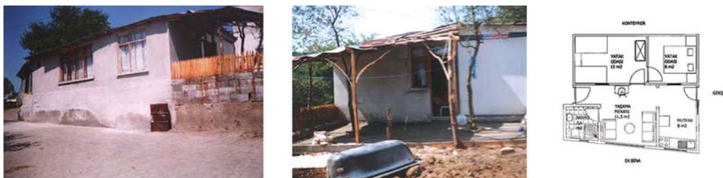
Figure 43 The self-built shelter by earthquake victims, combining the reprefabricated house with an extension.
