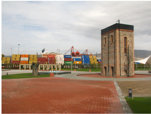
Figure B-10 The Restored Gas Factory in Alsancak
