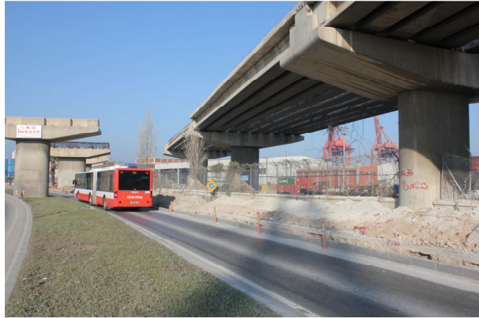
Figure 4-1 Recent Construction of the Viaduct towards the Port
