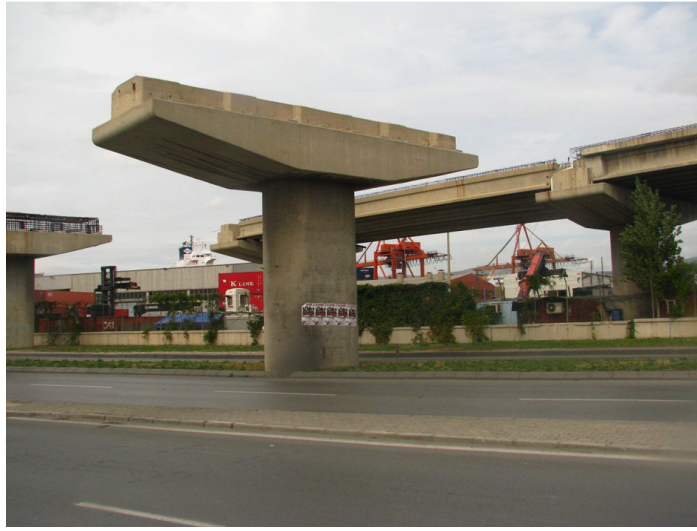
Figure 1-1 Incomplete Viaduct of Izmir-Çeşme Highway
