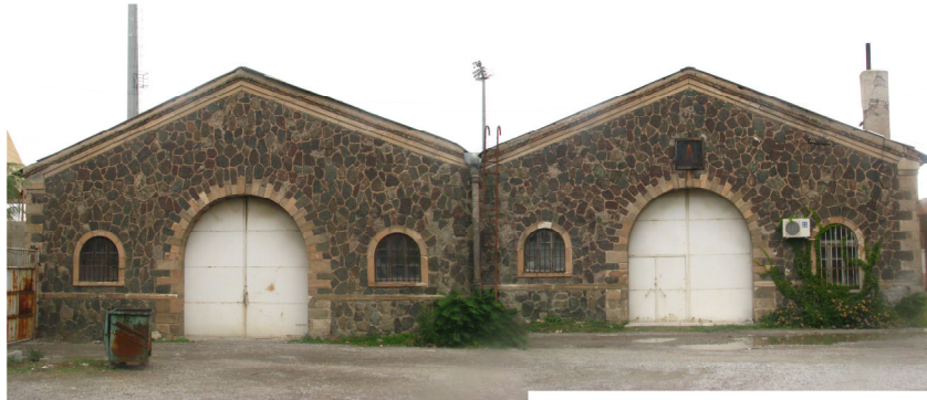
Figure B-2 Two of the Annexes of Alsancak Train Station
