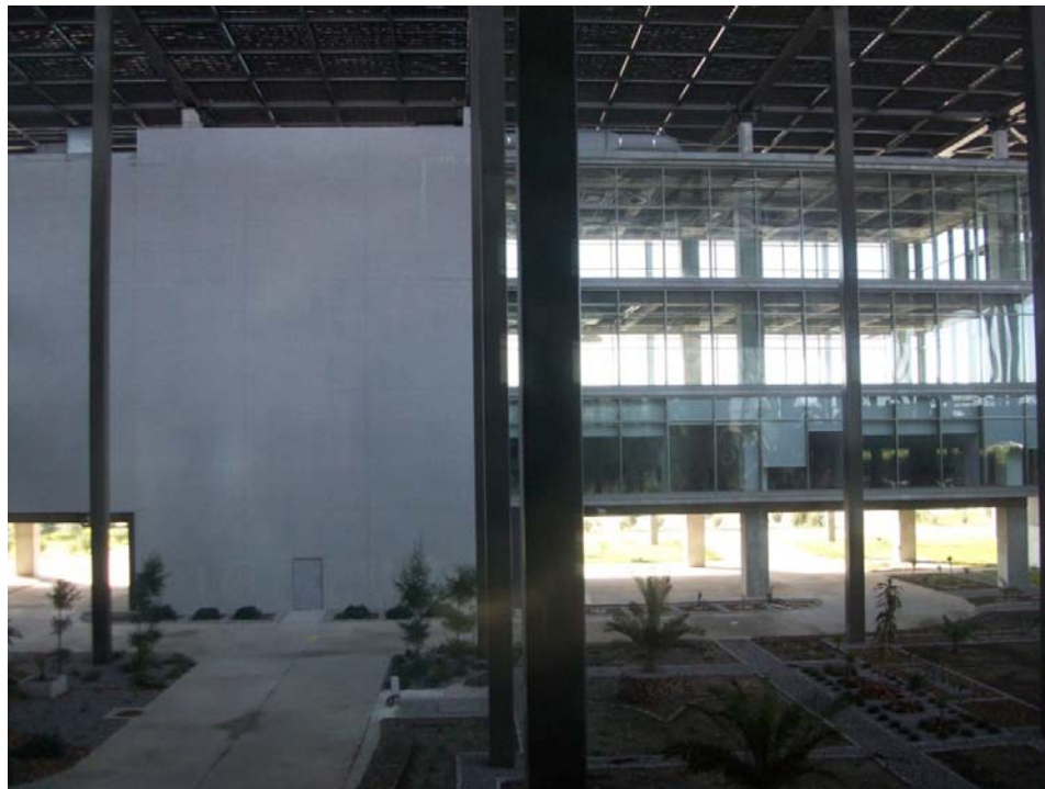
Figure 4.3. Three Floor Building Which Was Left Empty For 3 Years
