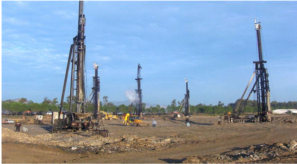
Figure 4.4. Soil Improvements Activities at Dalaman Airport.
