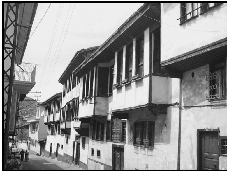
Fig. 69 Bey Street Houses (in a row)
