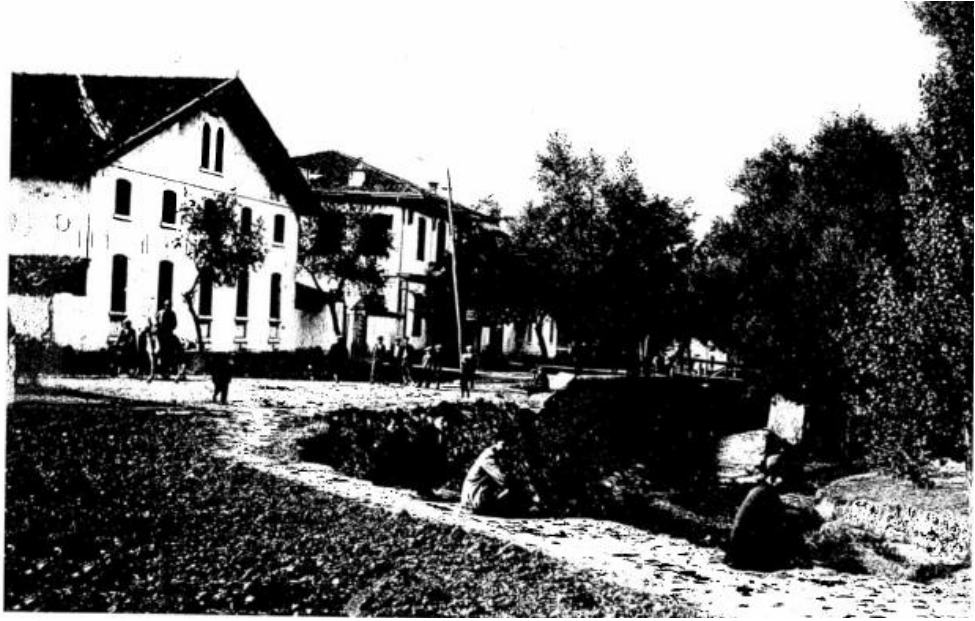
Fig. 32 Reji İdaresi Building (1930)
