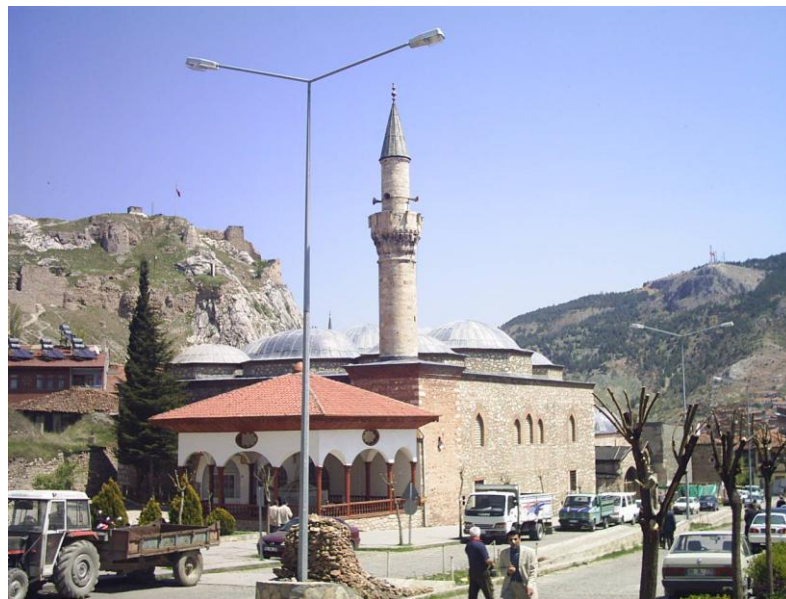
Fig. 8 Takyeciler Mosque attached to the Bedesten
