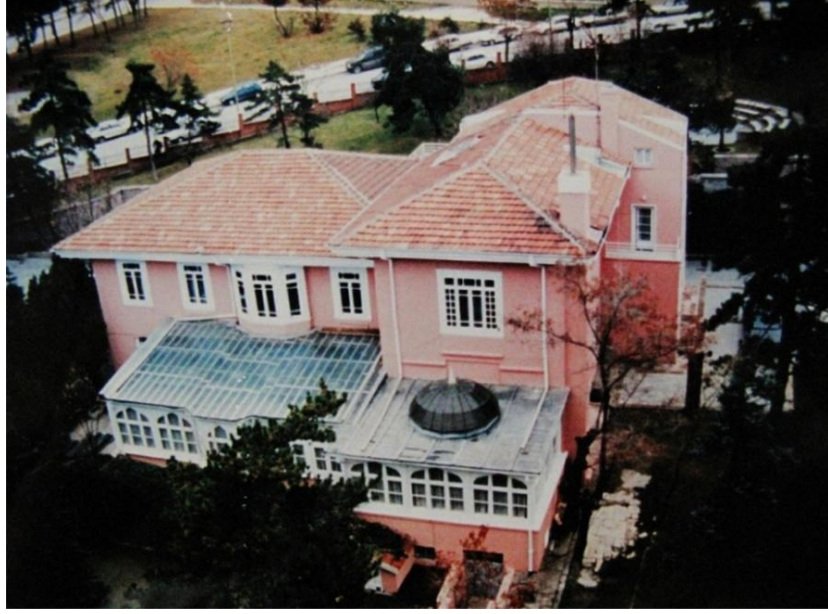
Fig. 13 İsmet İnönü House (Pembe Köşk) with its extensions (ballroom at the front and dining room at the right) 138
