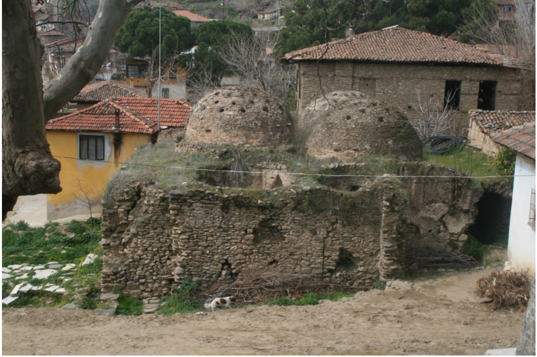
Figure 9, South Facade of Çukur Hamam
