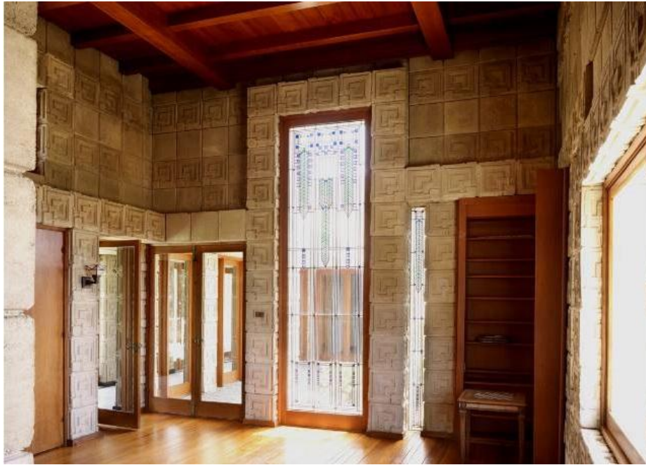
Figure 1. Frank Lloyd Wright textile blocks, Ennis House, Los Angeles Source: http://takesunset.com/2010/02/frank-lloyd-wright-ennis-house-2607-glendower/ [Last accessed August 21, 2011]
