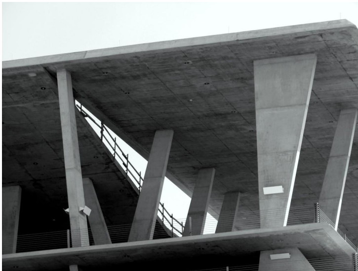
Figure 30. Parking Garage columns and slabs
