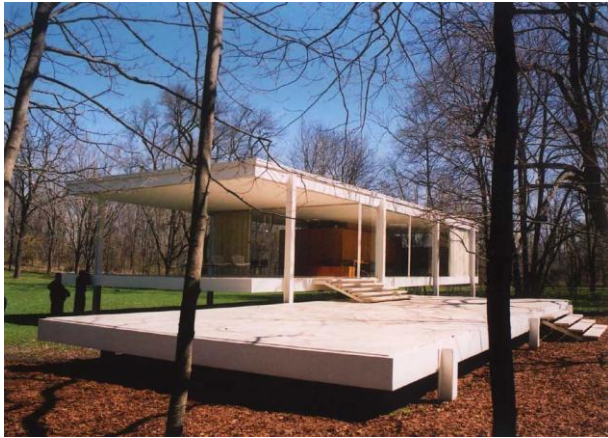
Figure 42. Mies van der Rohe's Farnsworth House
