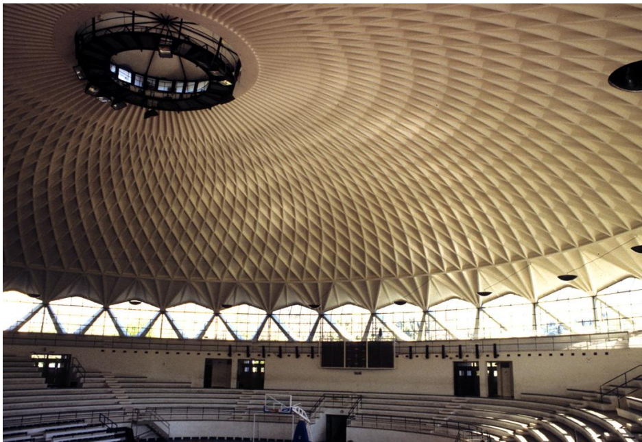
Figure 5. Pier Luigi Nervi, Small Sports Palace, Rome, structural detail
