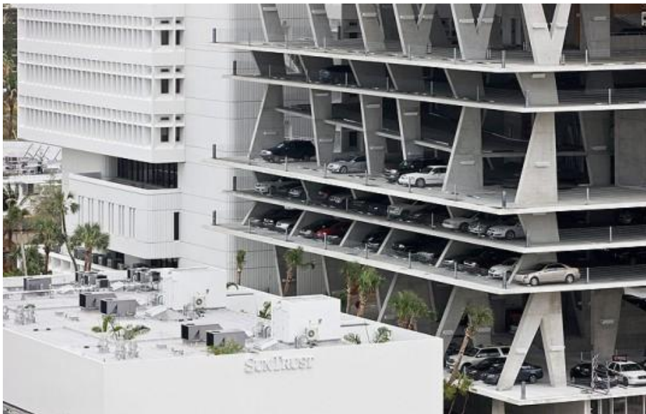
Figure 28. Parking Garage and existing Sun Trust building
