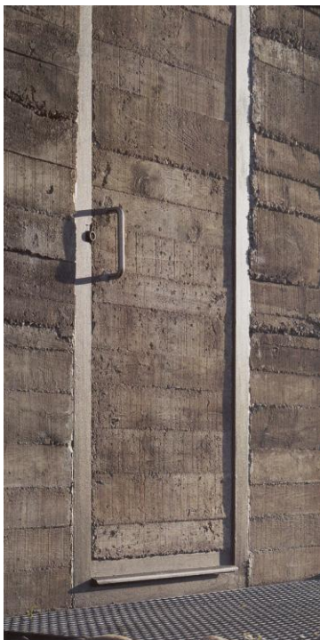
Figure 41. De Blas House outside of the concrete box, door detail
