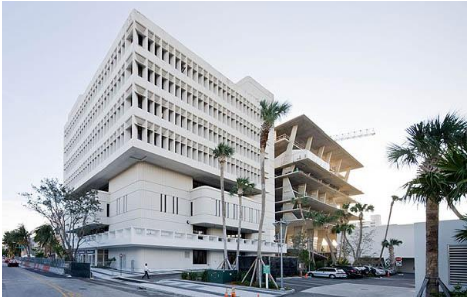
Figure 27. Parking Garage and existing Sun Trust building
