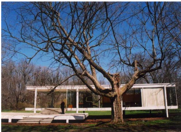
Figure 43. Mies van der Rohe's Farnsworth House
