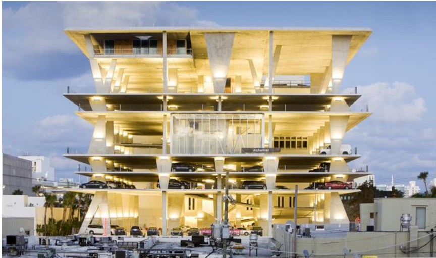
Figure 31. Parking Garage, lighting structure
