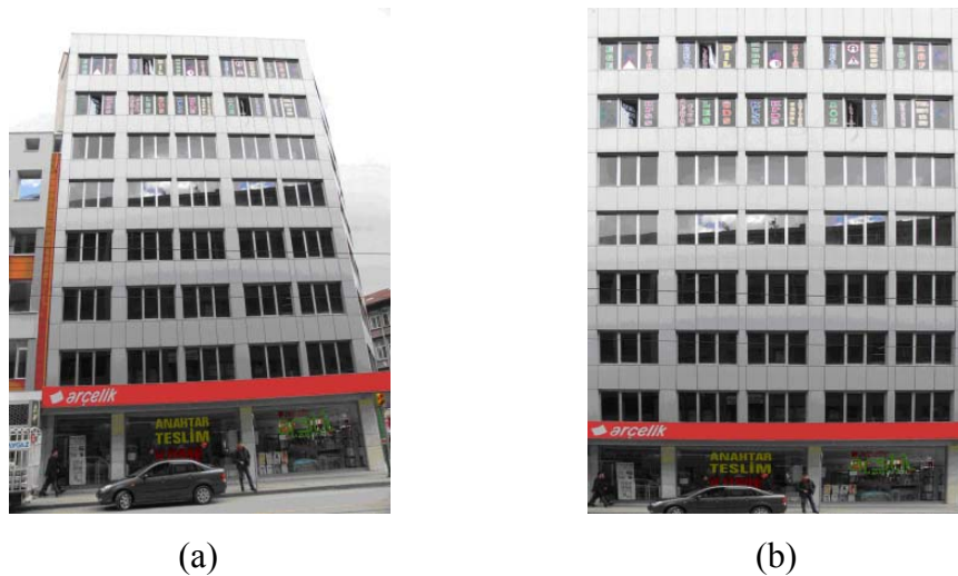
Figure 5.4. (a) Before and (b) after image rectification of an example façade image from the study area
