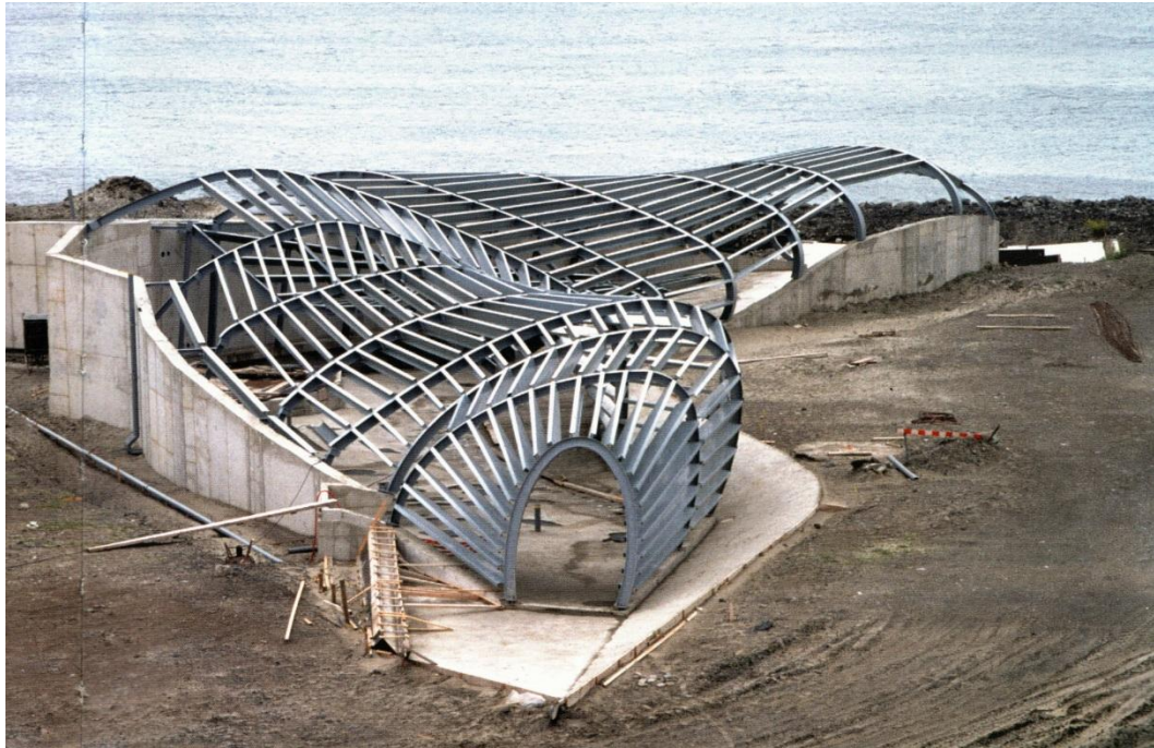
Figure 4.31 Structural frame of HtwoOexpo, primary curved frames and secondary straight beams, Lars Spuybroek/NOX Architects Source: Ibid. 23.
