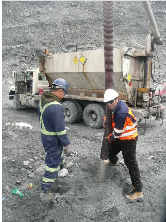
Figure 2.4 Loading blasthole with ANFO bulk truck
