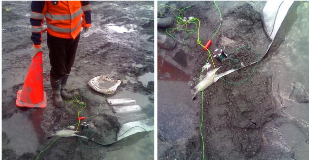
Figure 4.4 Wet hole loaded by bulk ANFO
