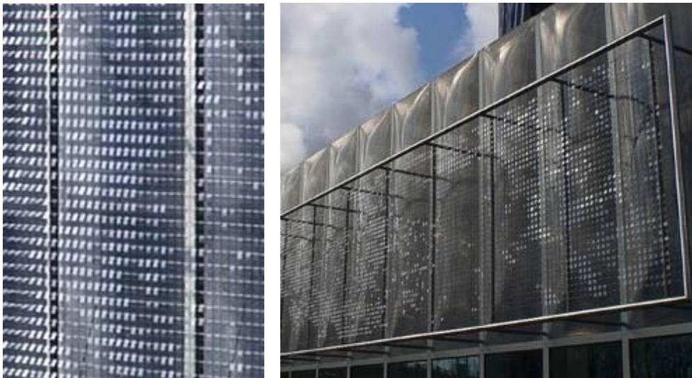
Figure 1: Wind responsive facade is design by Cepezed in collaboration with Ned Kahn Studios and constructed in 2008 in Netherlands.
