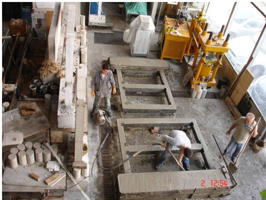
**Figure 3.1.** Vibration of Frame Concrete in Formwork
