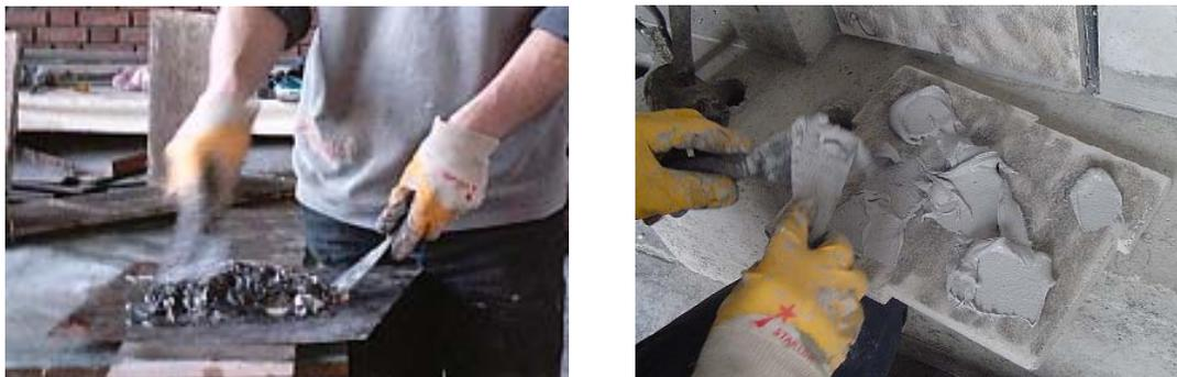
**Figure 3.7.** Sikadur – 31 Epoxy Mortar Preparations
