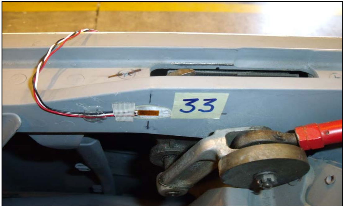
Figure 3.5.2: Linear strain gauge on longeron inner flange at the near of its cut-out
