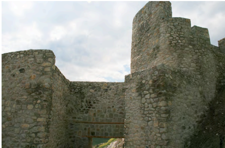
Figure 3 Restorated southern walls of the castle
