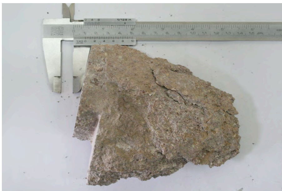
Figure 10 Deteriorated and flaked surface of Stone 4
