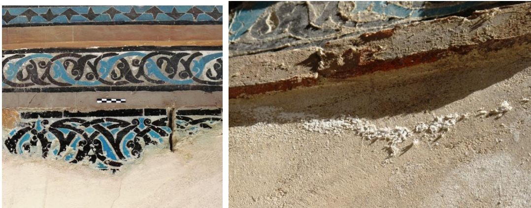
Figure 3.1 North Eyvan wall and dome. New restoration material was in contact with the original tiles and florescence was seen
