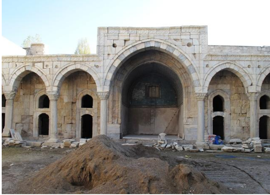
Figure 2.2 General view of Sivas Gök Medrese (2011)
