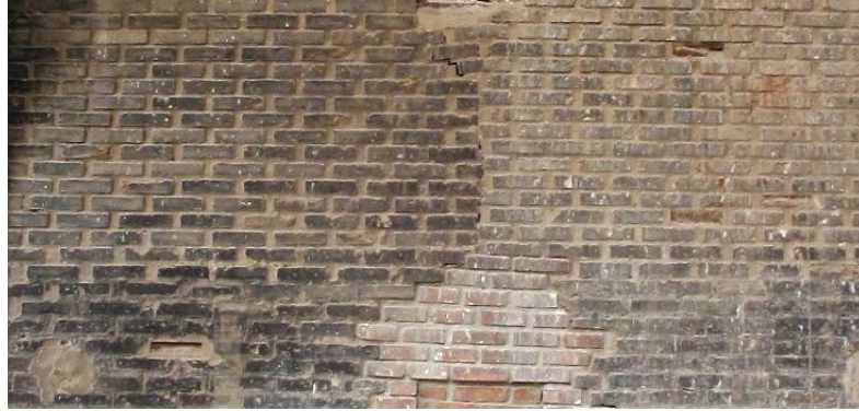
Figure 1.1 Brick units at the interior side of Sivas Keykavus Hospital (Daruşşifa), 2010
