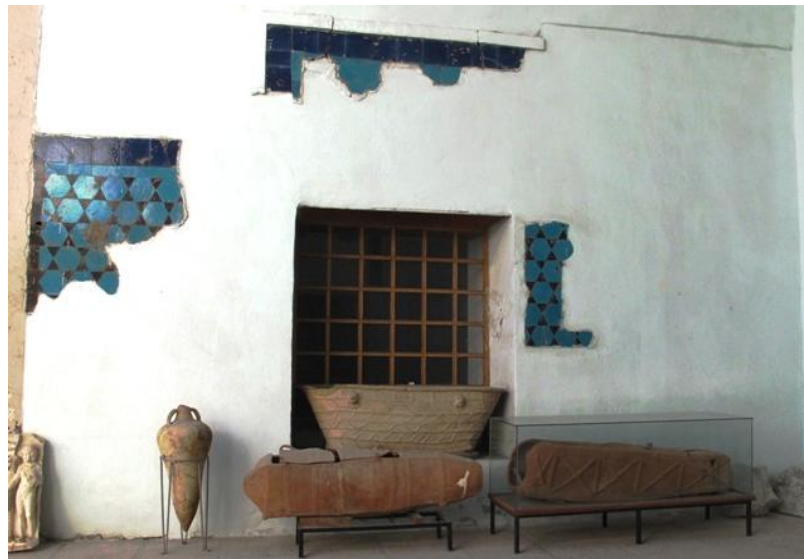
Figure 2.6 Left wall of main eyvan. Plain ceramic tiles were mostly lost (2011).
