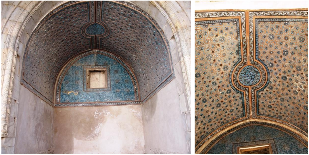
Figure 2.3 General view of South Eyvan; Sivas Gök Medrese (2011)
