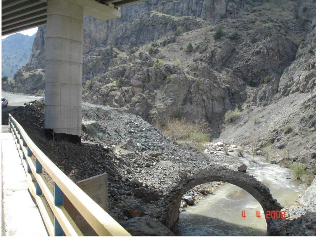
Figure 4.13 Pier of Kırkgeçit 7 Viaduct and Historical Bridge
