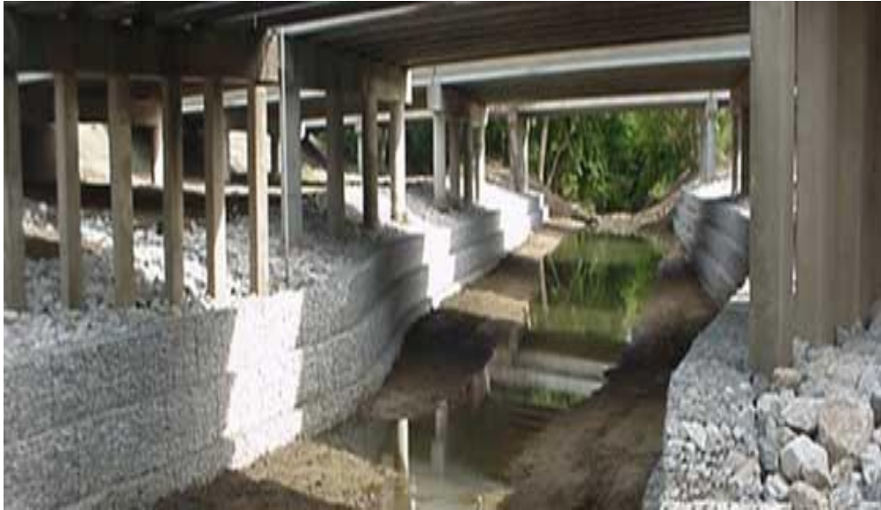
Figure 3.11 Use of Gabion Boxes around Bridge Piers
