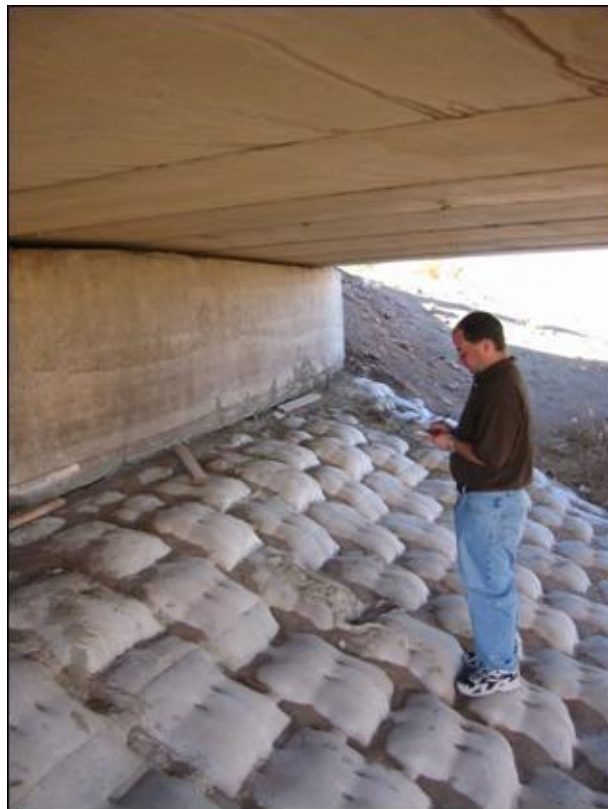
Figure 3.13 Typical Grout Filled Mattresses (FHWA, 1989)
