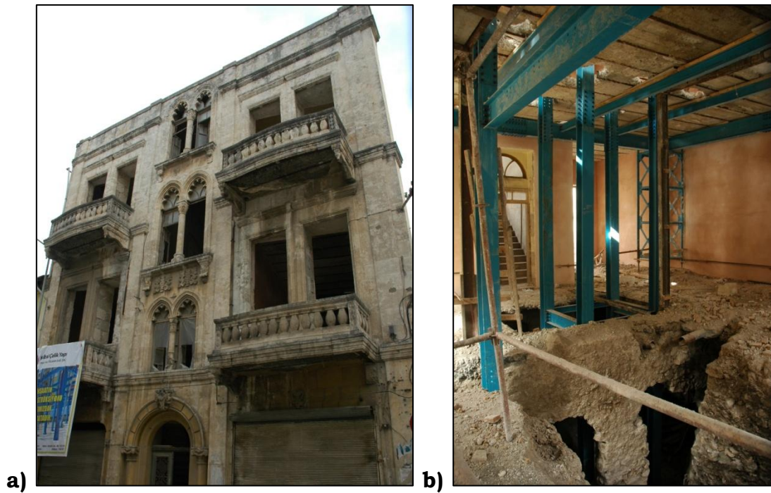
Figure 3.50. a) A neo-classic French Mandate Period building (Photograph: Rifaioğlu, M.N., 2007). b) Inappropriate intervention to convert a building into a hotel, which caused deteriorations to the original floors and ceilings of the building (Photograph: Rifaioğlu, M.N., 2007).
