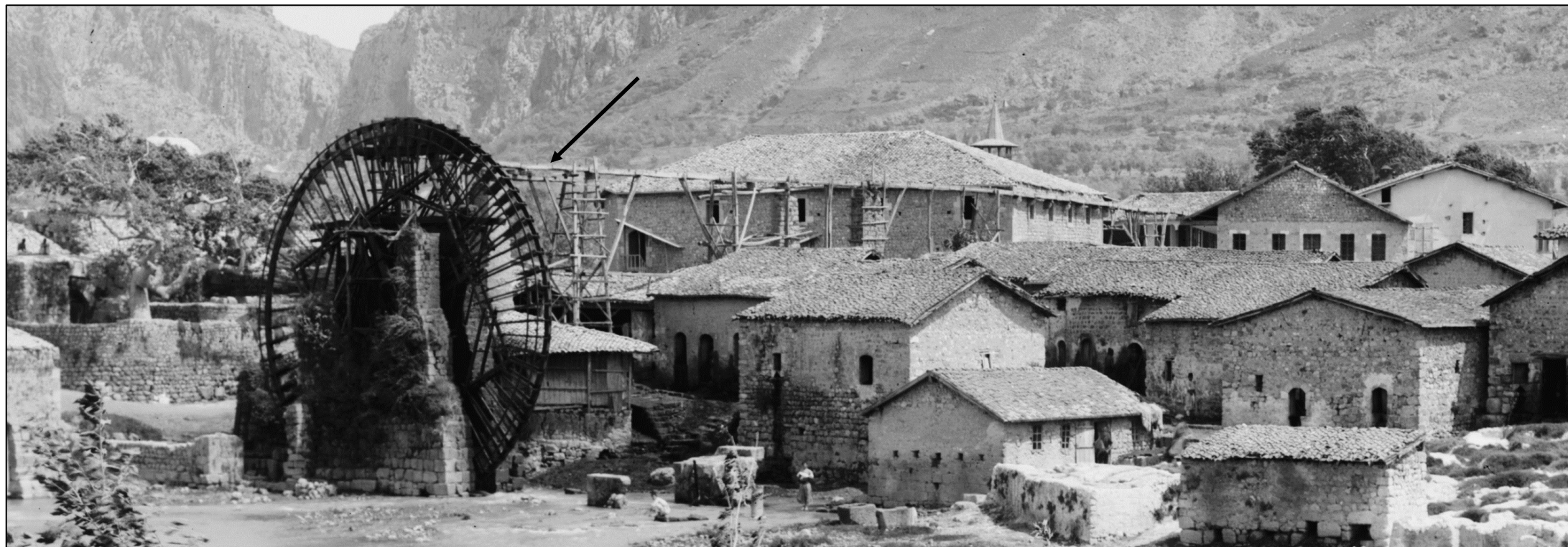
Figure 3.9. The Nauras along the banks of Asi River which carried water to the historical urban core (Source: Library of Congress)
