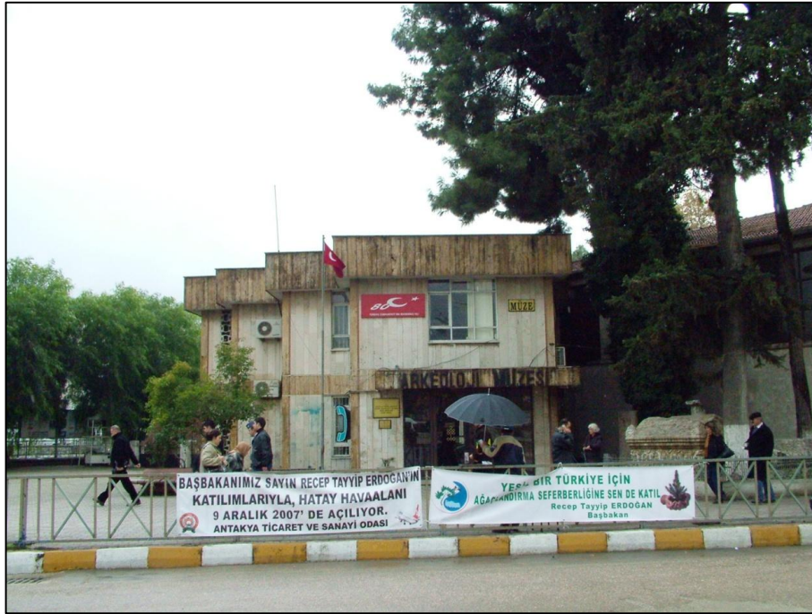
Figure 3.33. The Archaeological Museum of Antakya, showing the later annex entrance (Photo taken by Rifaioğlu, M.N., 2007).
