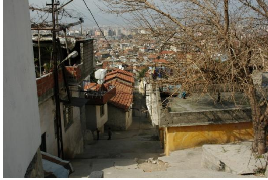
Figure 3.56. The current status of the physical characteristics of the urban transformation area (Photograph: Rifaioğlu, M.N., 2010).
