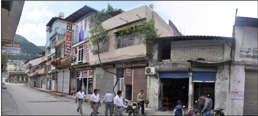
Figure 3.59. The light industrial workshops (Photograph: Rifaioğlu, M.N., 2010).
