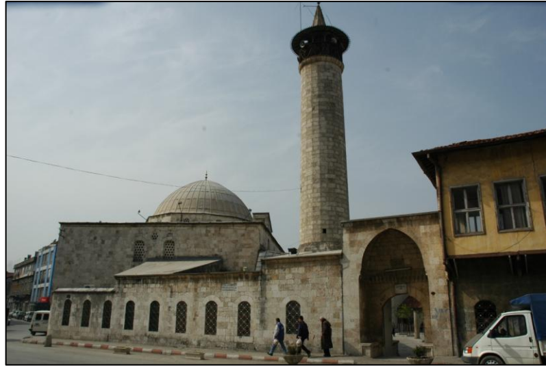
Figure 3.58. Habib Neccar Mosque and its surroundings (Photograph: Rifaioglu, M.N., 2010).
