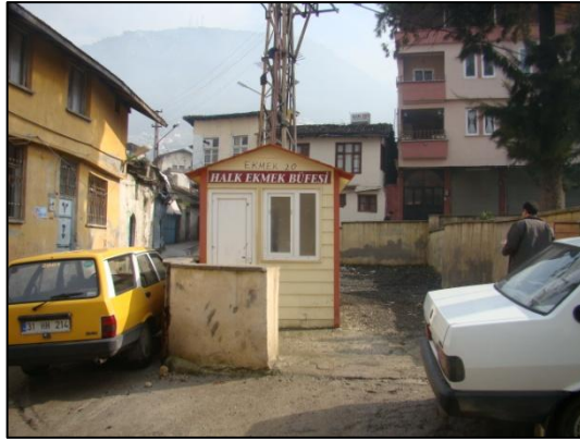
Figure 4.104. The Public Bread kiosk on the site of the bakeries that existed in 1929 (Photo: Rifaioğlu, M. N., 2009)
