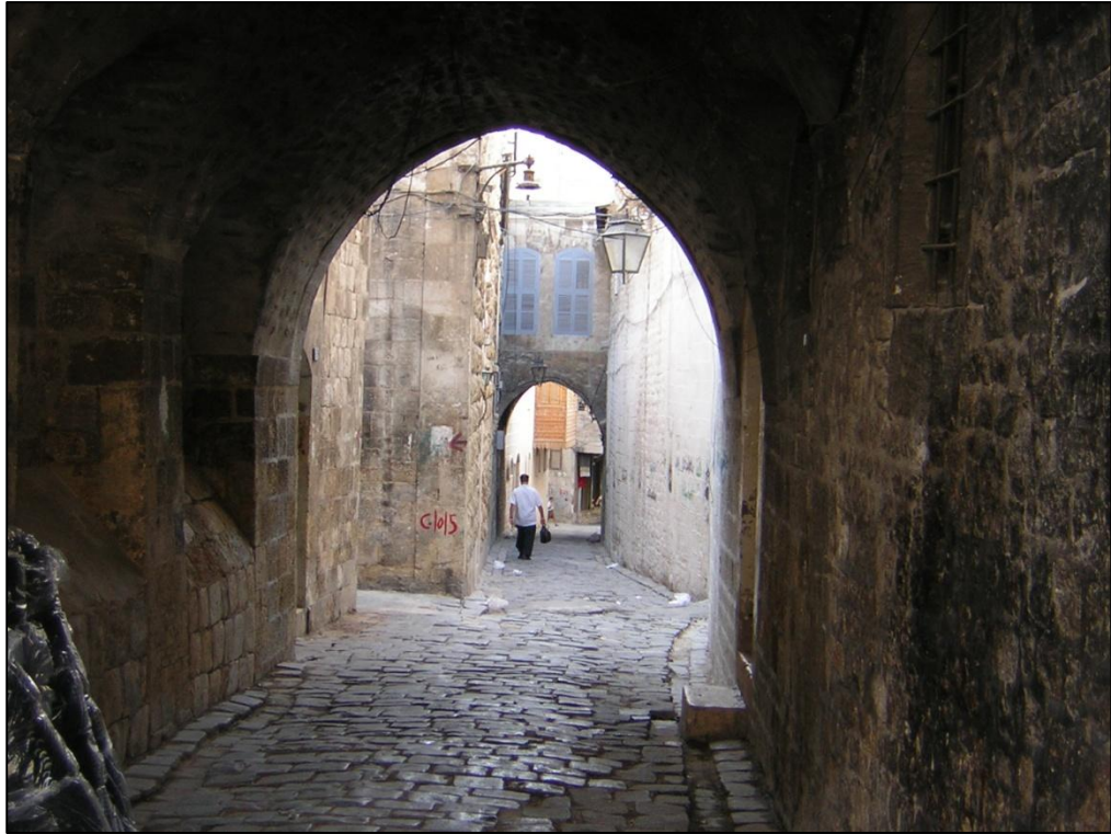
Figure 2.8. Sabat over a public street in Aleppo (Photograph taken by Rifaioğlu M.N., 2005).
