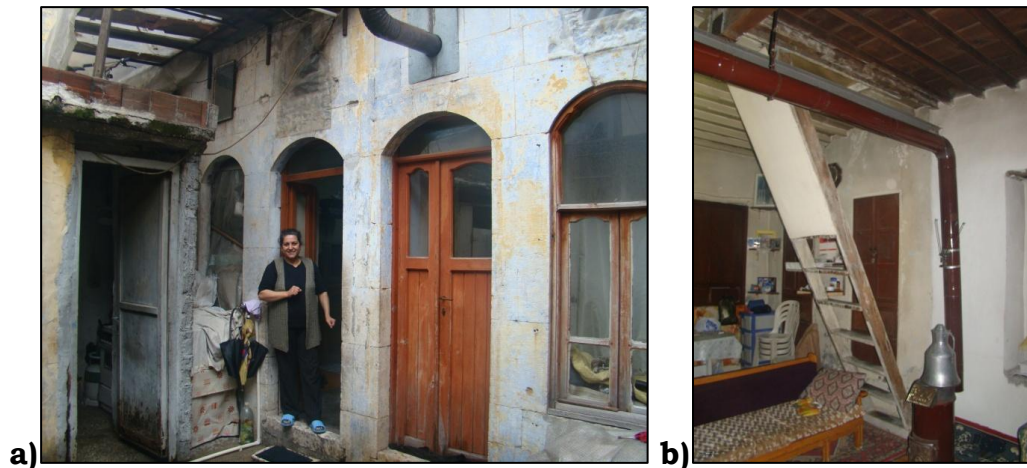
Figure 4.97. a) Two adjacent one-room dwellings located next to an Alewite visitation. b) The dwellings have been modified with a later addition of an upper floor (Photos: Rifaioğlu, M. N., 2009)
