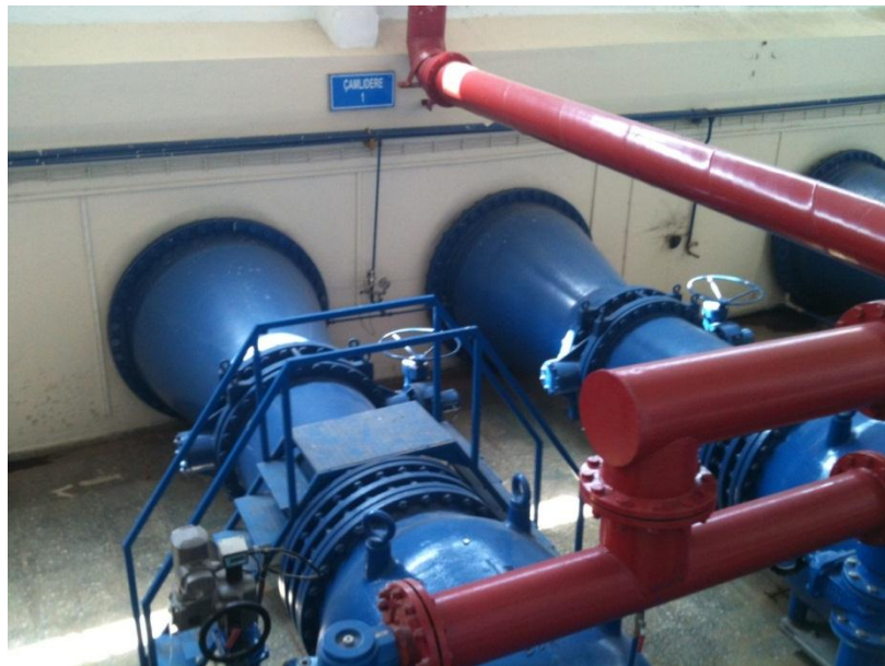
Figure E.3 Çamlıdere 1 pipeline entrance
