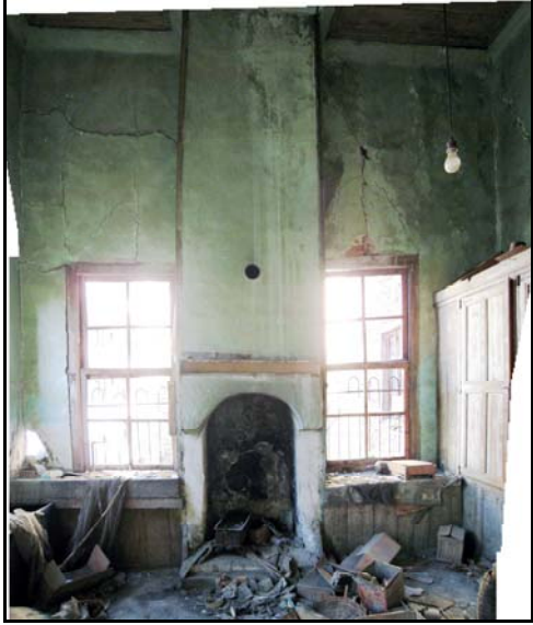
Figure 2.38. East Wall of Space 105
