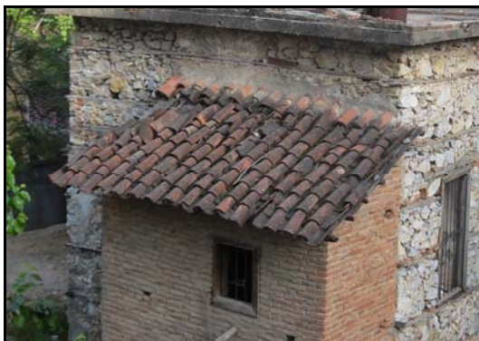
Figure 2.67. The roof of WC mass a- view from outside
