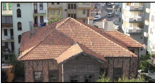
Figure 2.61. The roof of the building a view from outside
