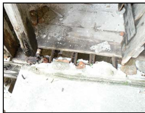
Figure 2.76. Concrete slab in staircase S02
