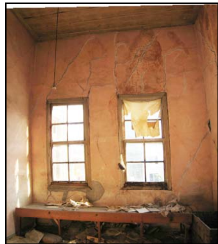
Figure 2.37. South Wall of Space 102
