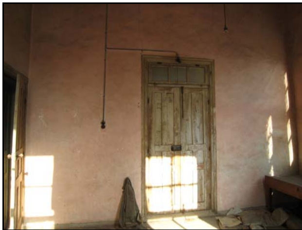
Figure 2.36. East Wall of Space 102
