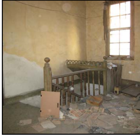
Figure 2.78. Stair railing in Space 101
