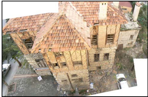
Figure 2.9. East facade of the building
