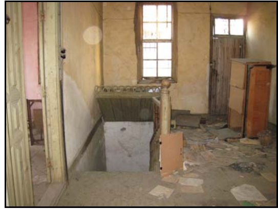
Figure 2.35. North Wall of Space 101
