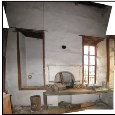
Figure 2.21. North Wall of Space E06
