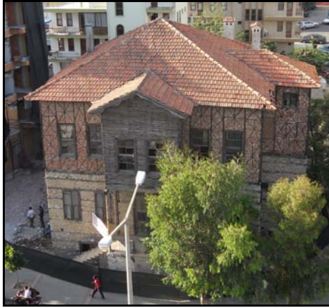
Figure 2.6. South facade of the building
