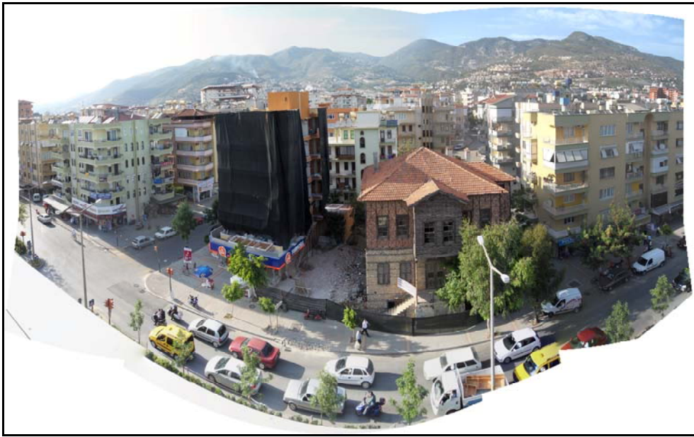
Figure 2.5. A General View of the Building
