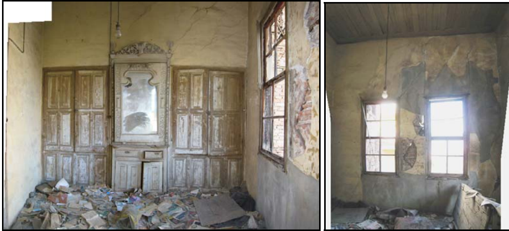
Figure 2.42. North Wall of Space 109 Figure 2.43. East Wall of Space 109
