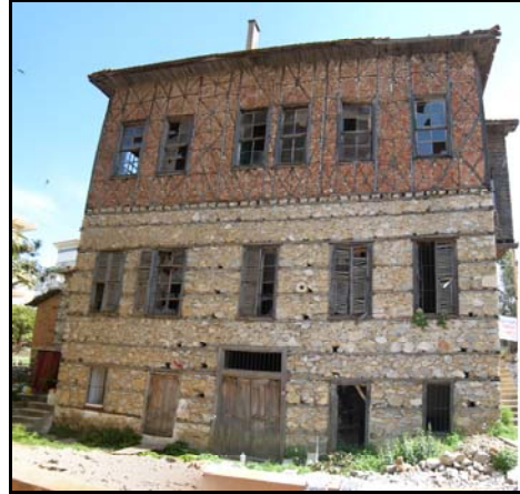
Figure 2.7. West facade of the building
