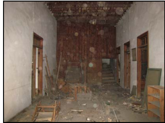
Figure 2.15. North Wall of Space E01
