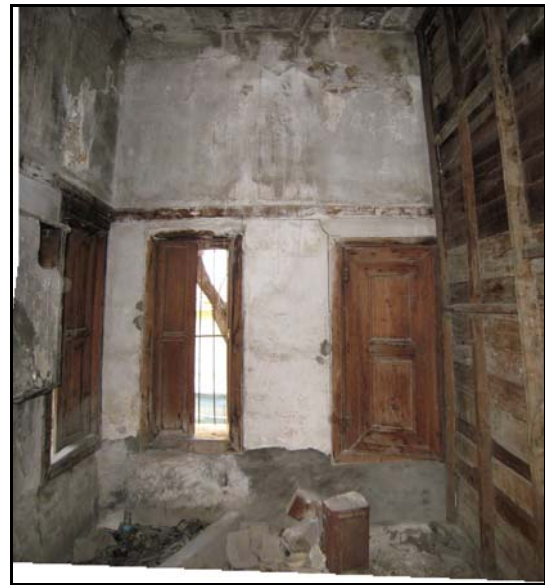
Figure 2.29. East Wall of Space E16
