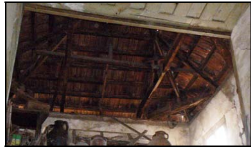
Figure 2.62. A view from inside from roof
