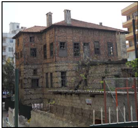
Figure 2.8. North facade of the building
