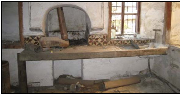
Figure 2.84. Kitchen counter in space E06
