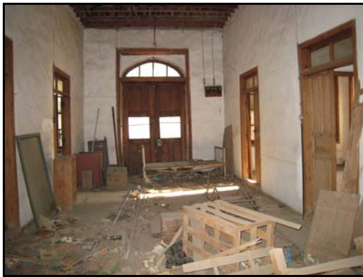
Figure 2.14. South Wall of Space E01
