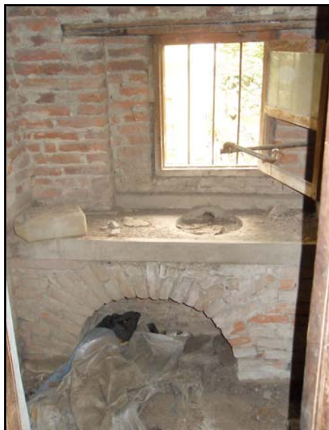
Figure 2.30. North Wall of Space E17
