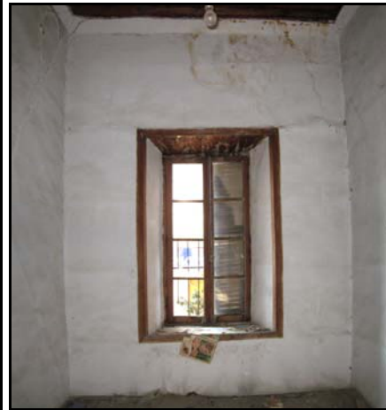
Figure 2.18. West Wall of Space E03
