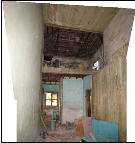
Figure 2.40. East Wall of Space 106
