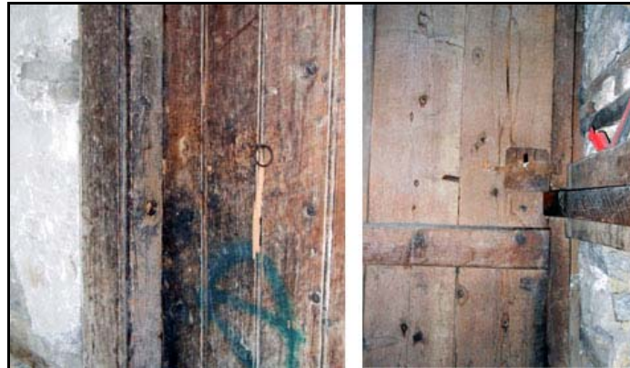
Figure A.2. “Tıraka” system on door D04
