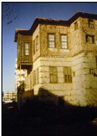
Figure D.4 Photographs submitted with the report dated 1990 (Alanya Museum Archive) (Continued)
