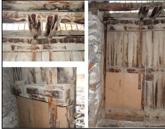
Figure A.1 “Tıraka” system on door D01
