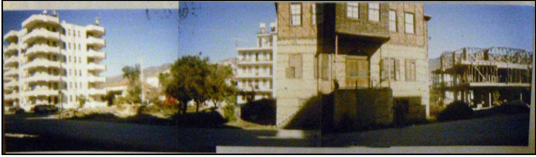
Figure 3.10. General view of the building in 1990 ( Alanya Museum Archive )
