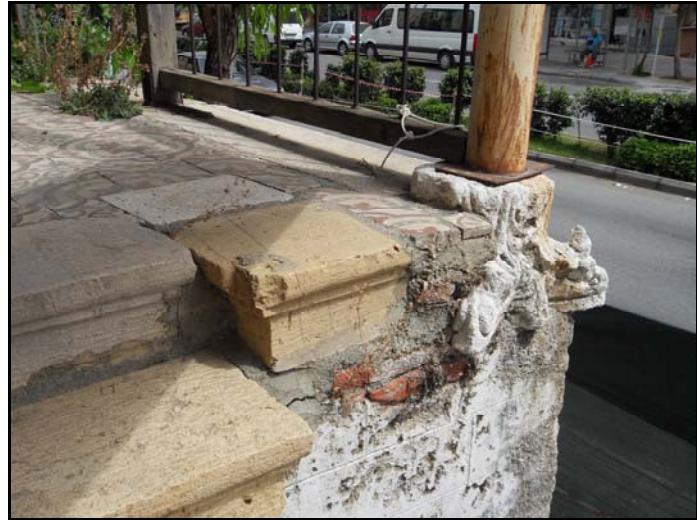
Figure 2.74. Reused materials in staircase S01
