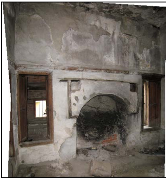
Figure 2.28. North Wall of Space E16
