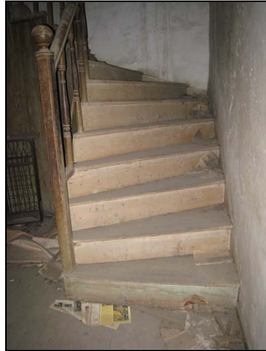
Figure 2.20. Timber Staircase in Space E05
