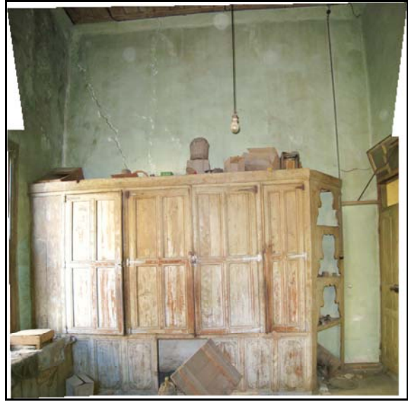
Figure 2.39. South Wall of Space 105
