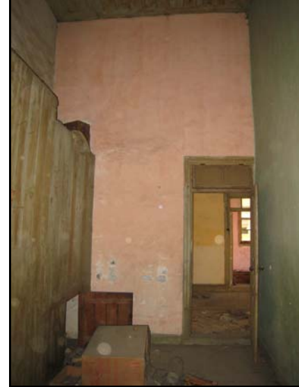
Figure 2.41. West Wall of Space 106
