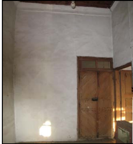
Figure 2.17. East Wall of Space E03
