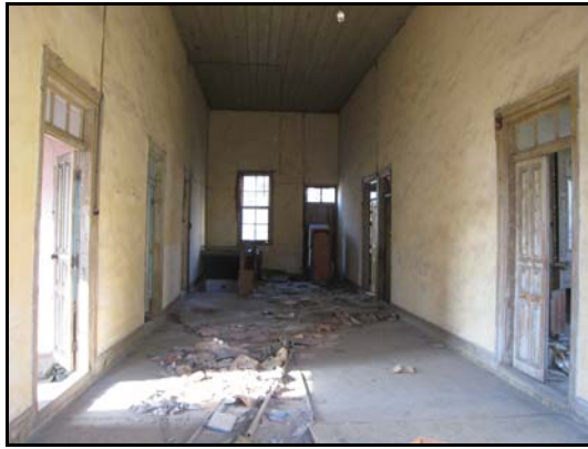
Figure 2.34. South Wall of Space 101
