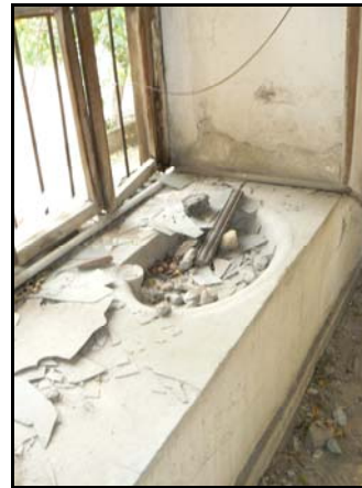
Figure 2.24. Lavatory in Space E07
