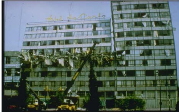
Figure 1.1: A picture of a hotel building that has a collapsed middle floor due to the impacts of September, 19 1985 Mexico Earthquake (Photograph taken from: http://www.smate.wvu.edu/teched/geology/GeoHaz/eq-Mexico/eq-Mexico-08.jpg )
