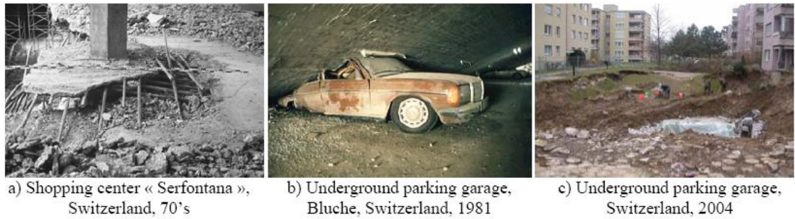
Figure 1.8 Punching Failures in Switzerland, (Mirzaei, 2010)
