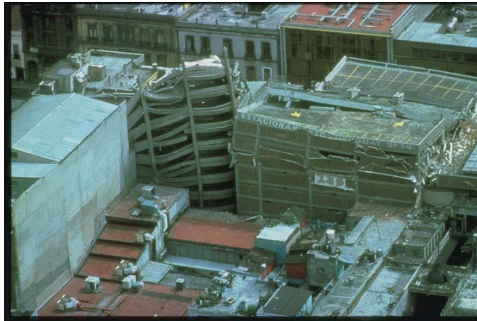
Figure 1.10 Example of collapse of waffle slab building failures in New Mexico (Rosenblueth, et al., 1986)
