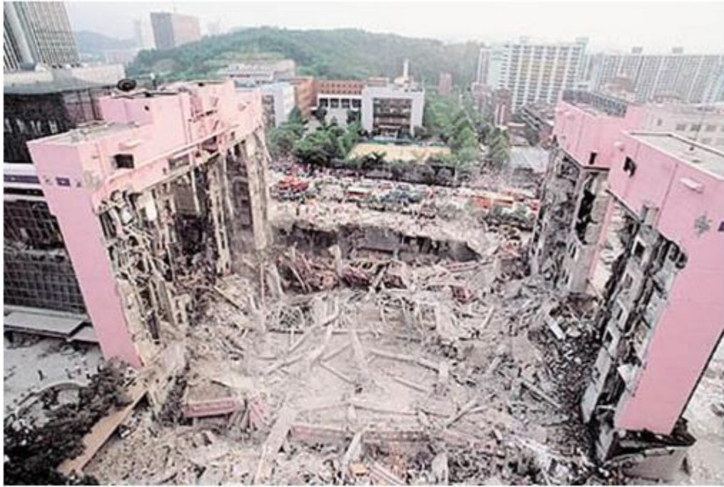
Figure 1.4 Sampoong Department Store after collapse, (Park T. W., 2011)
