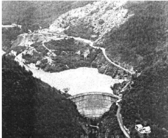
**Figure 3-2** - Picture of the Pontesei dam and artificial reservoir, the 1959 landslide is clearly visible in the upper part of the picture (Panizzo et al., 2005).
