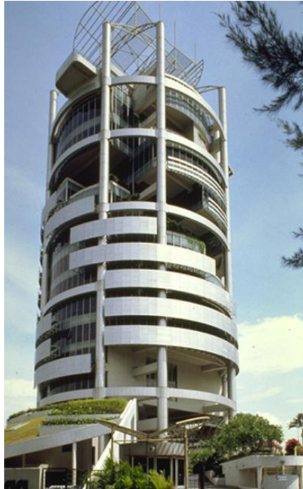
Figure 2.18. Menara Mesinaga, 1992, Kuala Lumpur (Source: Google Images)
