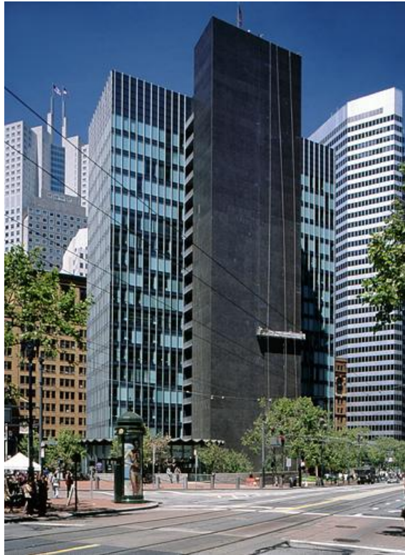
Figure 2.25. External view of One Bush Street, San Francisco (Source: Google Images)
