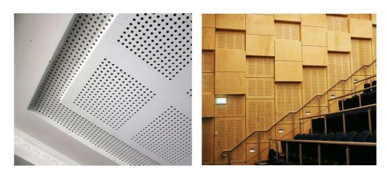
Figure 3.3 Resonant absorber examples
