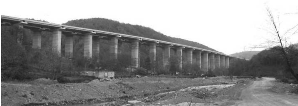
Figure 3.7 General view (from SW) of the Bolu viaducts (after Faccioli et al., 2002)
