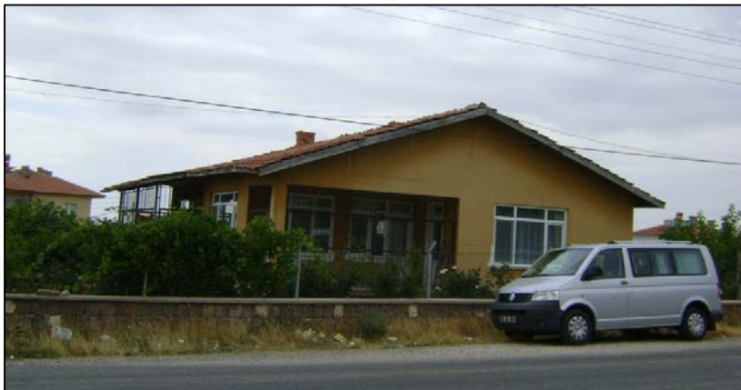
Photo 7: One of the Ulusoy residences outside mansion complex
