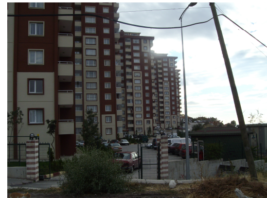
Figure 61: Large scale construction facilities of transformation in Şentepe (Çiğdemtepe)
