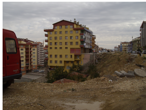
Figure 40: Apartments under the level of roads
