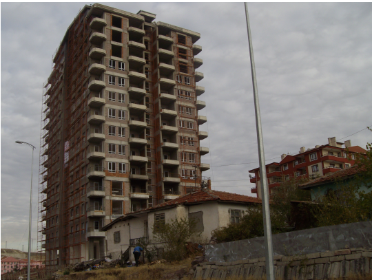
Figure 63: New construction facilities of transformation in Şentepe
