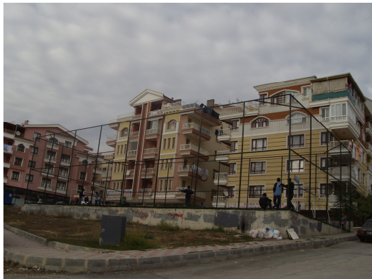
Figure 69: Finished sports areas
