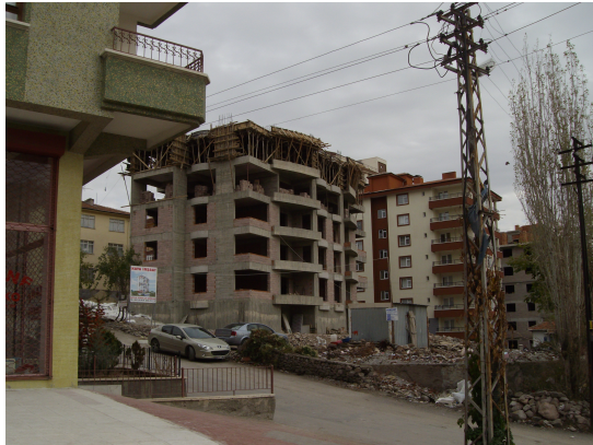
Figure 68: New constructed buildings and refuse materials of demolish and construction
