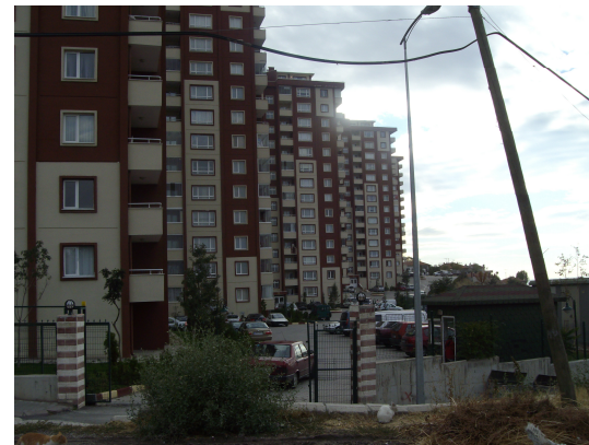
Figure 71: A 'gated community' with security guards
