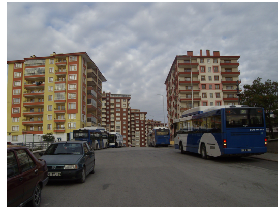
Figure 64: A Street composed of transformed buildings in Şentepe
