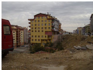
Figure 67: Squatters and refuse materials of demolish and construction are part of the landscape
