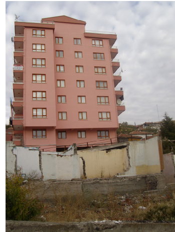
Figure 66: Demolished Dwellings in Şentepe
