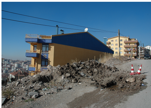
Figure 39: Apartments under the level of roads
