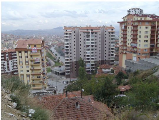
Figure 59: New construction facilities of transformation in Şentepe
