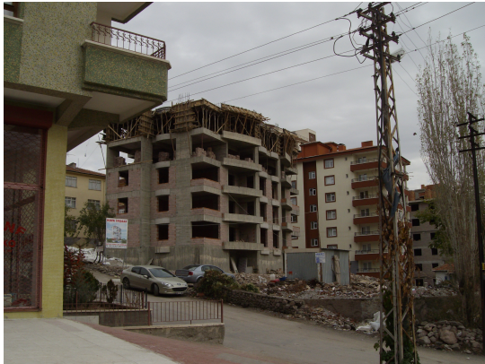
Figure 58: New construction facilities of transformation in Şentepe
