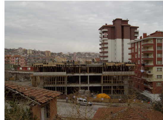
Figure 60: New construction facilities of transformation in Şentepe
