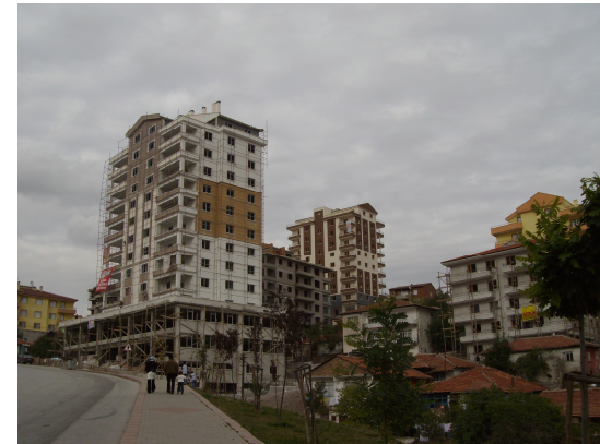
Figure 57: New construction facilities of transformation in Şentepe
