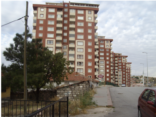
Figure 62: Large scale construction facilities of transformation in Şentepe (Çiğdemtepe Quarter)
