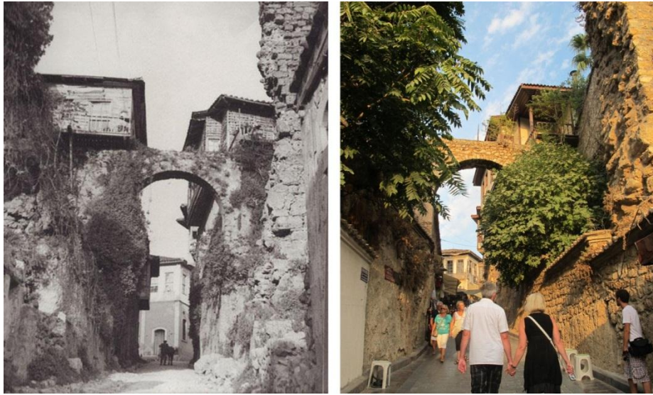
Figure 4.11 One of the gates of the port in 1953 and in 2012 (personal archive of Tazecan; personal archive)
