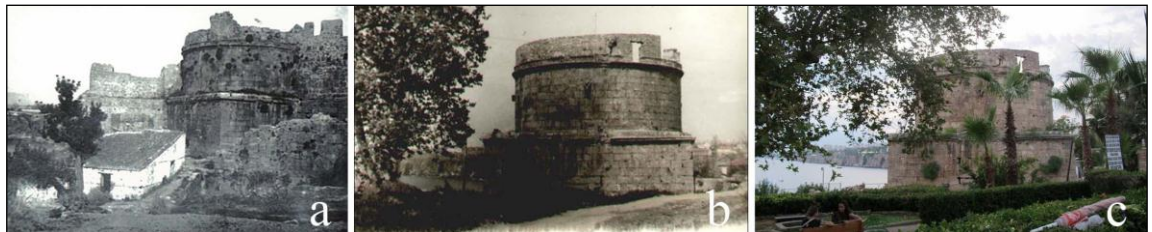
Figure 4.5 Hıdırlık Tower in (a) 19 th century, (b) after 1930s, (c) 2012 (Resource: (a) personal archive of Dündar; (b) personal archive of Tazecan; (c) personal archive)
