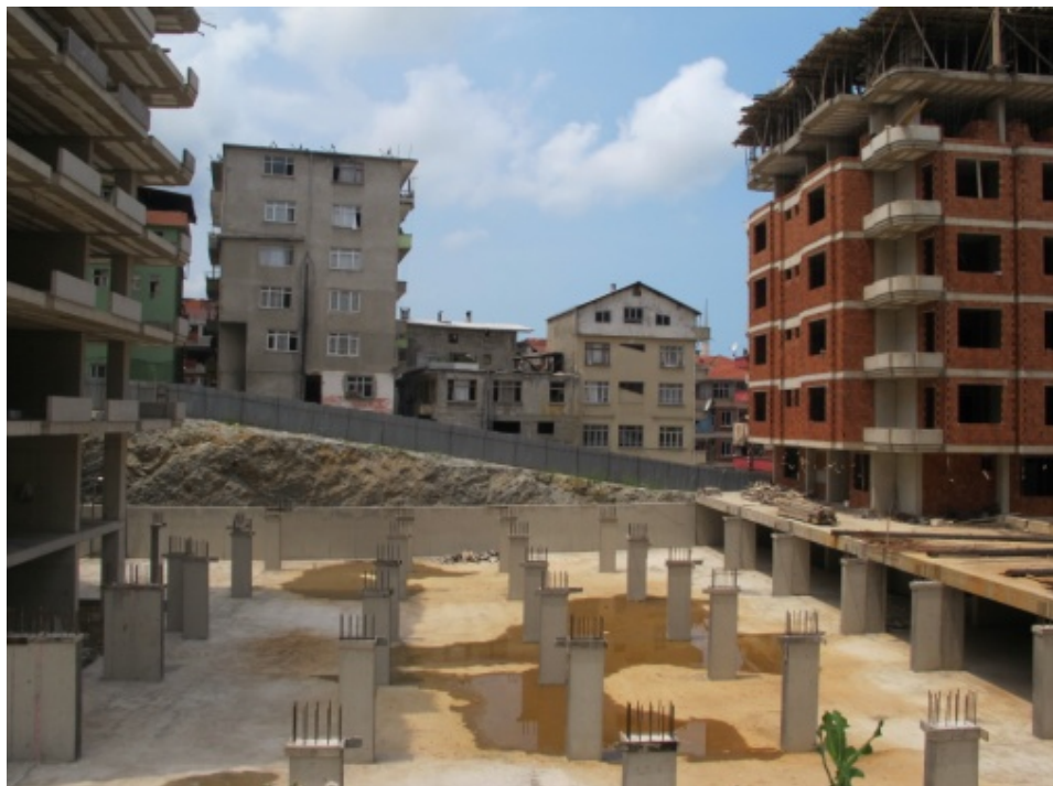
Figure 6-24 The same garden turns to construction site in 2012 (personal archive)
