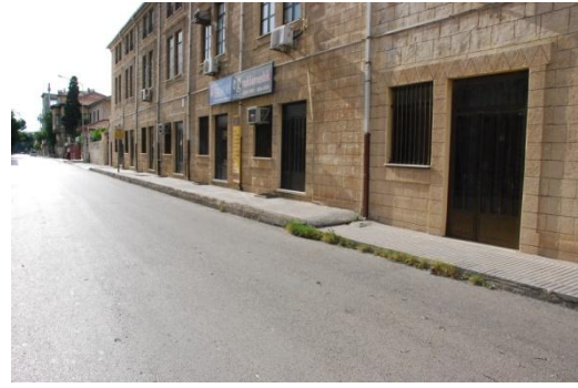
Deformed ramps and insufficient width of walking paths for wheelchair.
