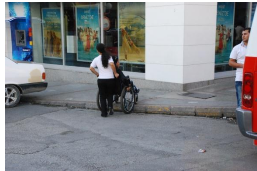
Over level between pedestrian way and traffic road, no ramp
