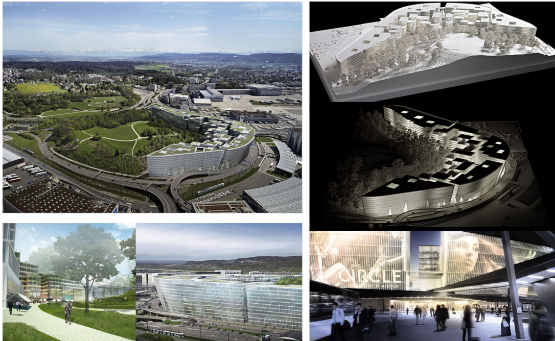
Figure 4.7: The Circle, at Zurich Airport, designed by Riken Yamamoto & Field Shop
