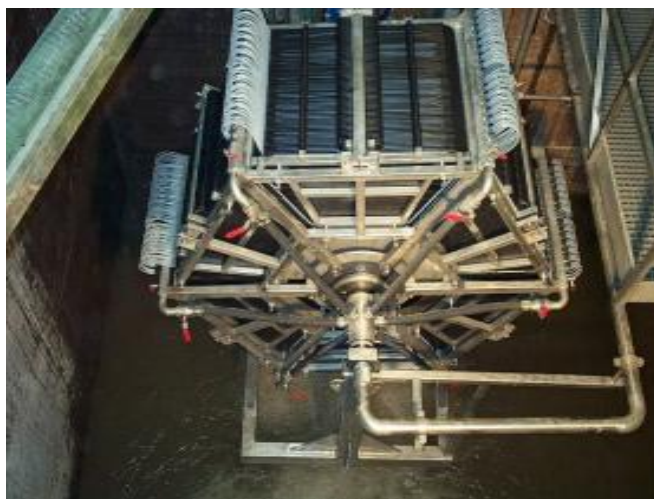
Figure 5: Vacuum Rotating Membrane System
