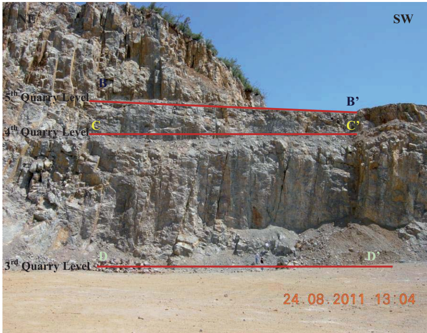
Figure 1.3. Different levels of the Gavurpinari limestone quarry and vertical layering of bentonite beds along the NE-SW direction
