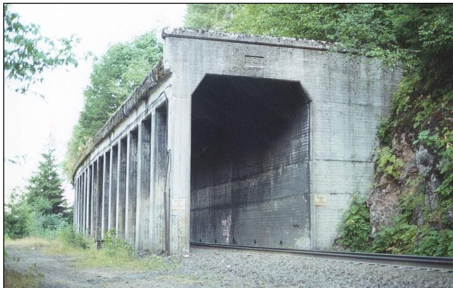
Figure 2.11 A rockshed structure constructed for a railway (Trainweb, 2000).
