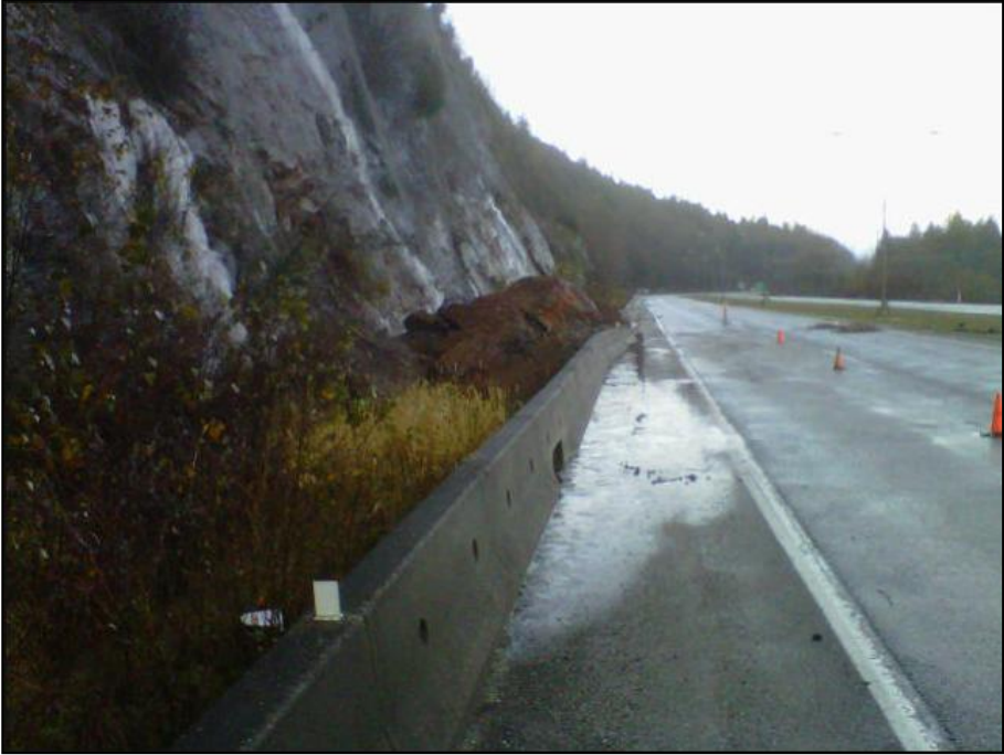
Figure 2.12 A ditch structure form a highway (TranBC, 2010).
