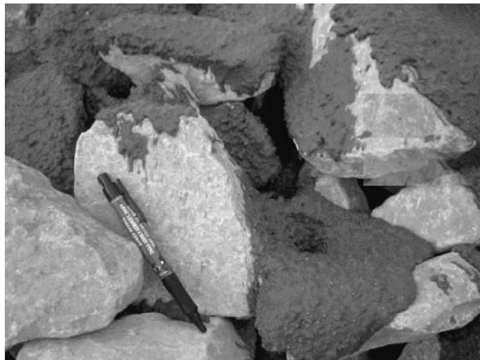
Figure 3.4 A typical view from and application of partially grouted (Lagasse et al., 2007)
