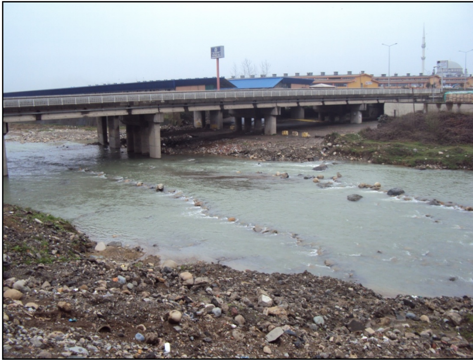
Figure 5.1 Upstream view of the bridge
